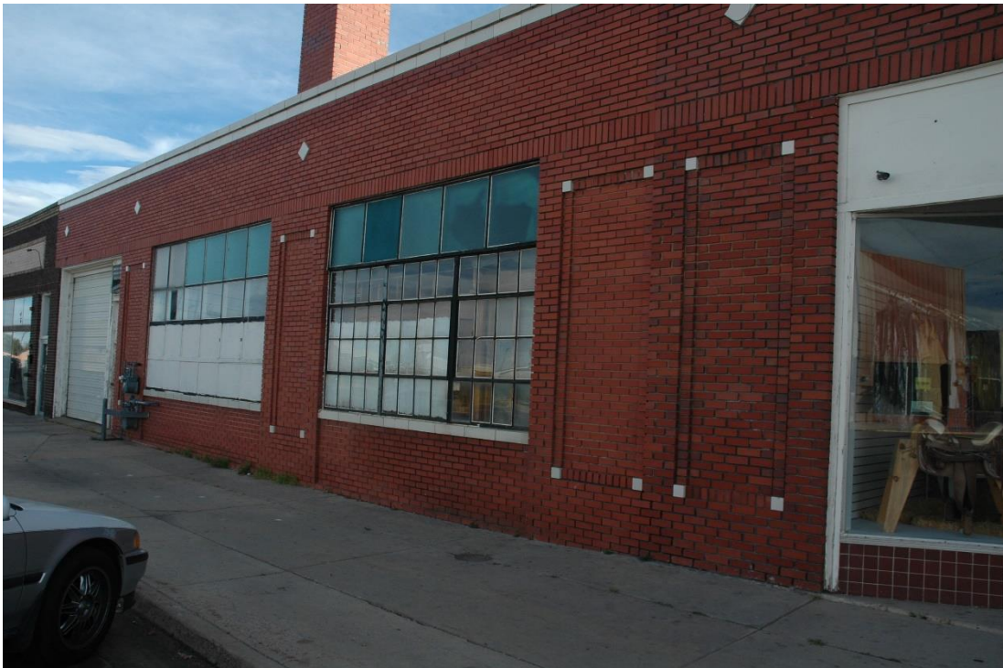
CD 1, Image 171, View to SE of north side
