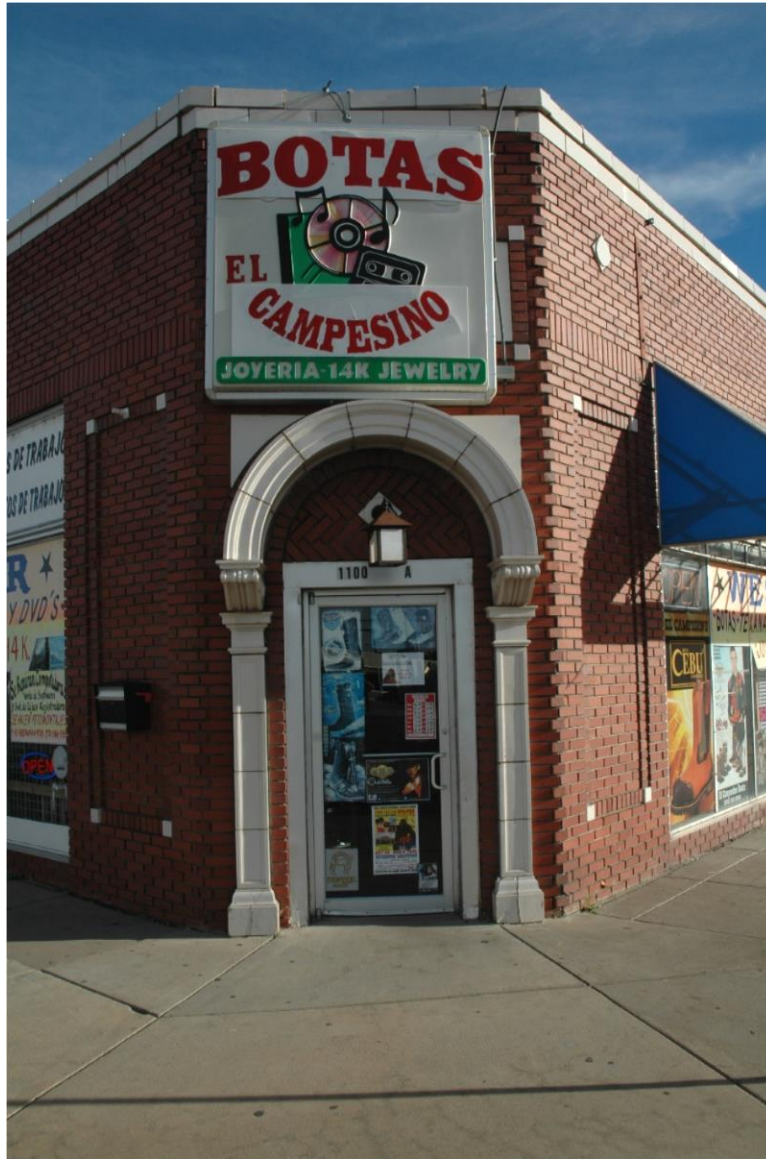
CD 1, Image 173, View to SE of corner entry
