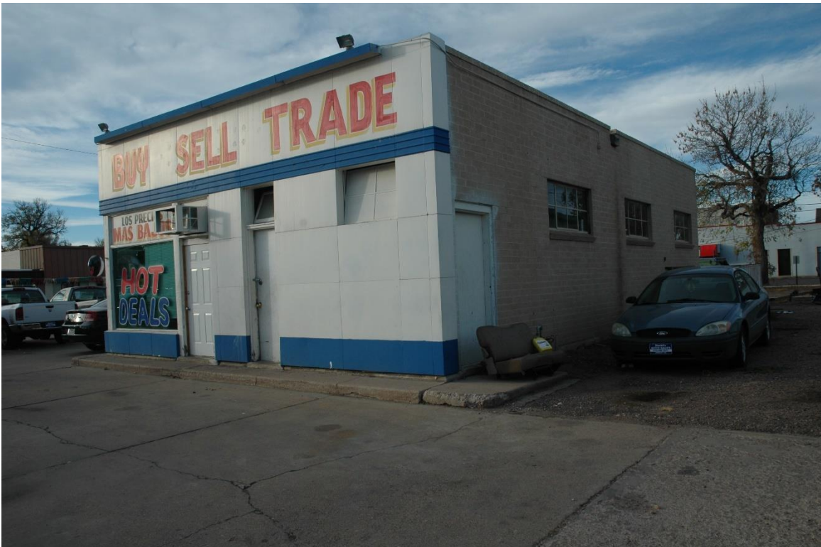
CD 1, Image 209, View to NW of south side and rear (east)
