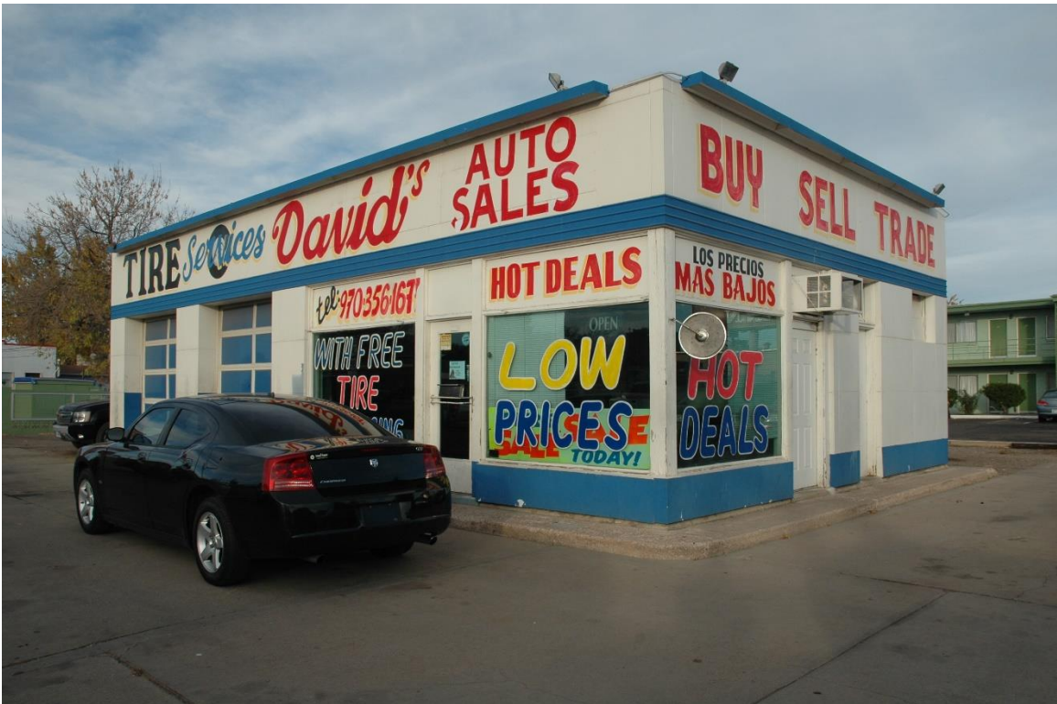
CD 1, Image 208, View to NE of façade (west) and south side
