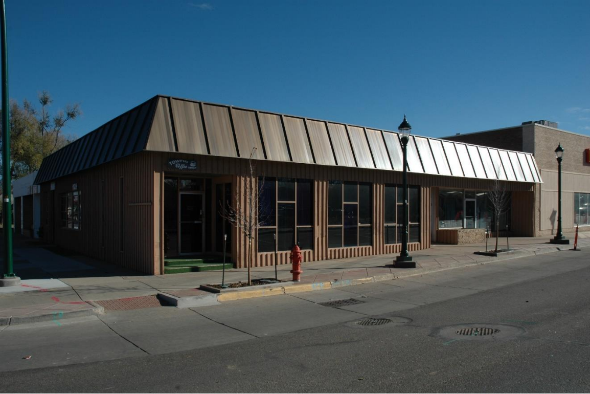
CD 2, Image 18, View to SE of façade (west) and north side
