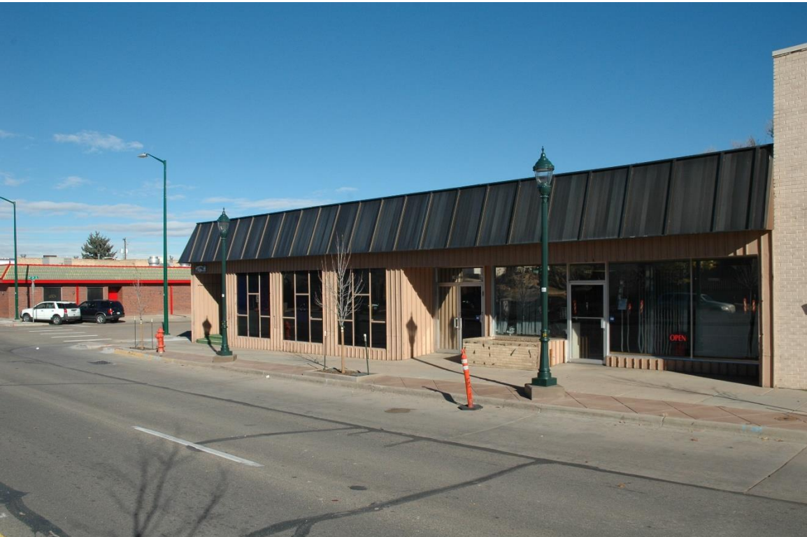
CD 1, Image 19, View to NE of façade (west)
