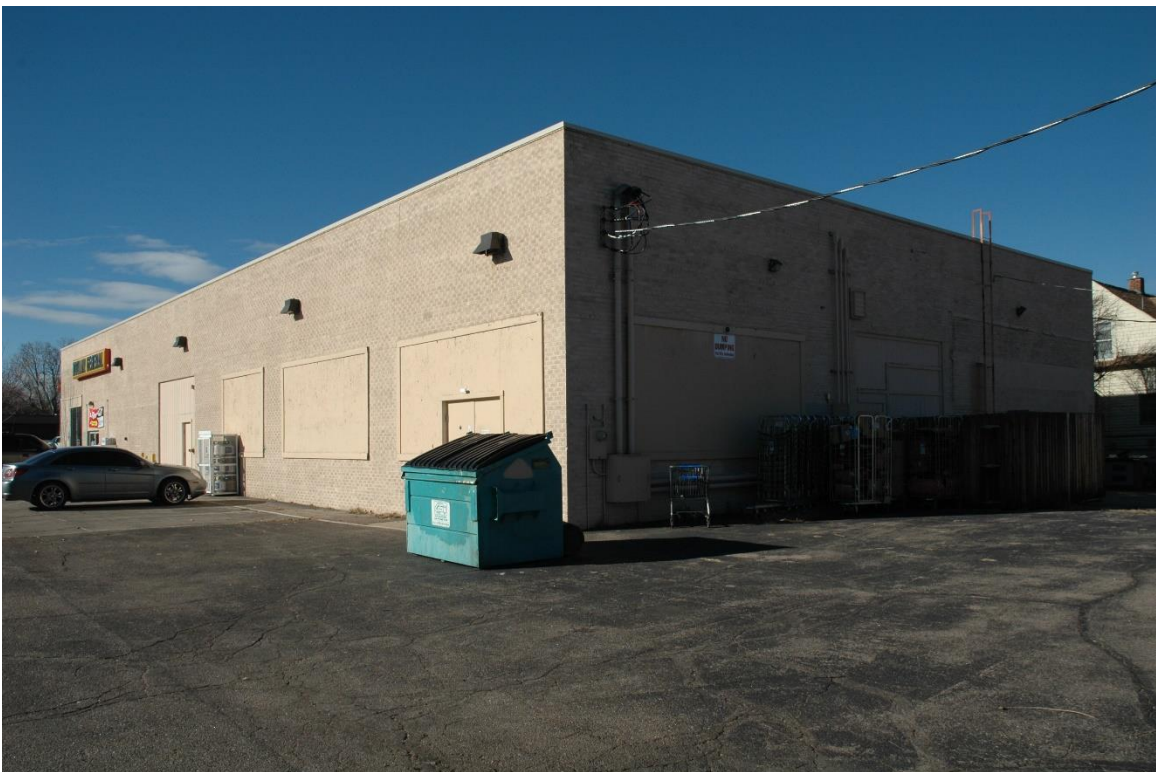
CD 2, Image 21, View to NW of rear (east) and south side
