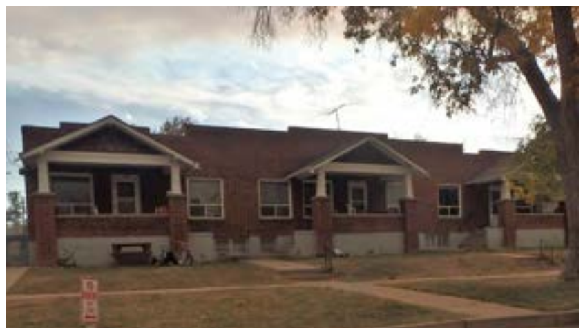
Figure 83. 1116-1120 17th Street. This three unit example of a terrace form is identifiable through its brick construction, parapet, and multi-unit façade.
