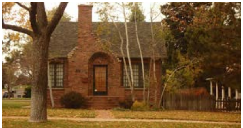
Figure 13. 1939 12th Avenue, looking west. Showing an example of the neighborhood's detached revivalist residences which are typically of moderate scale and possess uniform set backs from the sidewalk.
