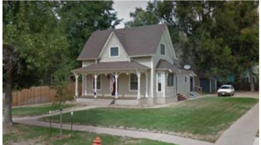
Figure 82. 1403 8th Street. The two room width and single room depth of this residence's main block shows its core to be that of an I-House. Assessor's data indicates this building dates to 1882.
