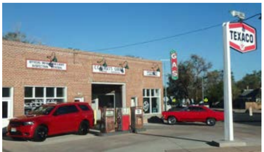
Figure 20. C.C. Kersey's Garage, 531 8th Street. This building shows the small-scale development prevalent throughout the Sunrise neighborhood which includes residential, commercial, and light industrial facilities.
