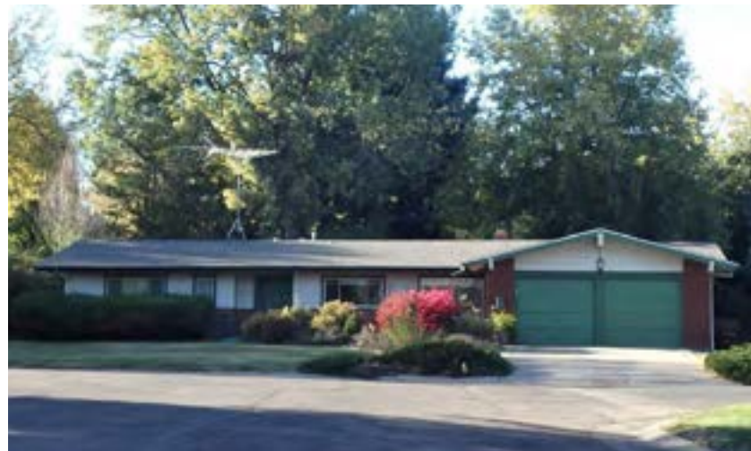
Figure 88. 2005 18th Avenue. This ranch style home is identifiable through its horizontal single-story form, its picture windows, and its attached garage. It is located in the pre-War Glenmere Park neighborhood and utilizes more traditional brick masonry and gable roofs.
