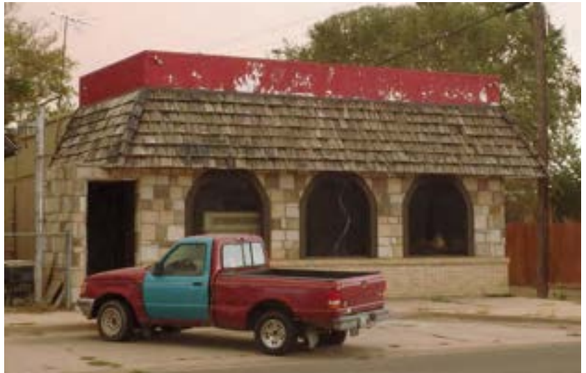
Figure 105. 1020 6th Avenue. Assessor's data indicates this building was constructed as a storage warehouse in 1963. The mansard roof, arched windows, and stone cladding all appear to be a later additions to modernize the building's primary façade for commercial usage.
