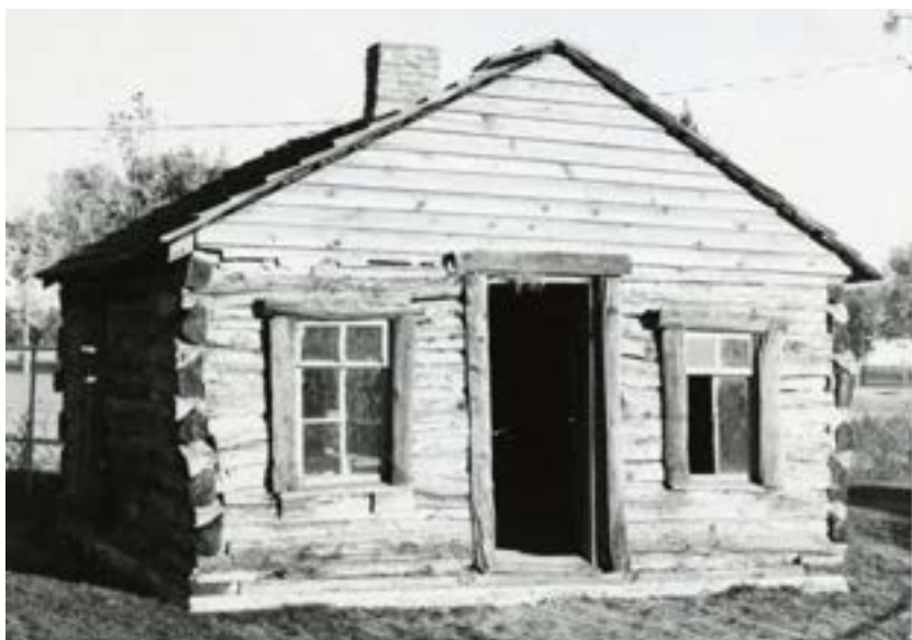
Figure 65. Original Weld County Courthouse constructed from hewn cottonwood logs with dovetail notching. This building was constructed around 1860 and relocated from its original site near Fort Vasquez in Platteville to Greeley's Centennial Village where it remains on display. AI-0464, City of Greeley Museums, Weld County Images Collection. 1979.
