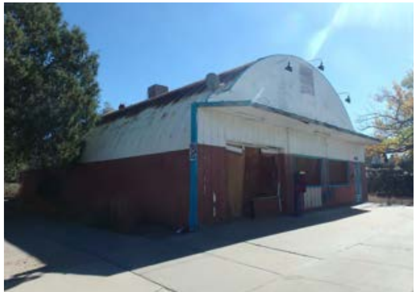
Figure 89. 402 11th Avenue. This Quonset hut has been adapted to a commercial purposes with a more traditional façade appended onto the huts original end. Its half-cylinder shape shows it to be an early example of the form.
