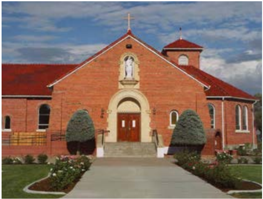
Figure 51. Our Lady of Peace Church, 1311 3rd Street (5WL.2577). This building possesses both architectural distinction as a good example of the Romanesque Revival style and ethnographic distinction as the house of worship for many Mexican immigrant Catholics who felt unwelcome at more established churches. It was determined field eligible for the NRHP in 1997 but needs to be resurveyed after a 2003 expansion. 2011.79.0006, City of Greeley Museums, Permanent Collection. N.d.
