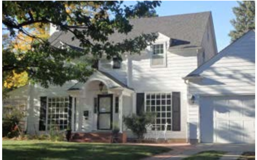
Figure 99. 1633 Glenmere Park Boulevard. This home is an example of Colonial Revival style, with its symmetrical, street-facing façade on a side-gable form, prominent central entry with classical detailing, multi-light sash windows, and shutters. Weld County assessor's data indicates it was constructed in 1941, making it a mature example of the style.
