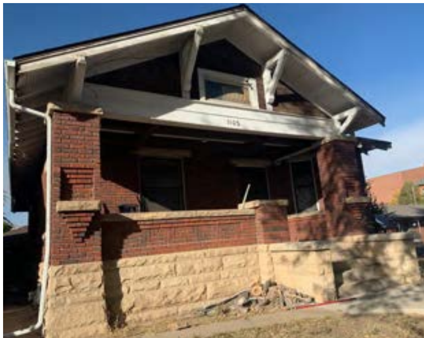
Figure 100. 1105 8th Street. Although this 1918 Craftsman residence employs elaborate materials including sandstone and an unusual textured brick, it exhibits hallmarks of the Craftsman style, including natural materials, heavy piers, exposed structural elements, and exposed eaves. Its expensive materials and unusual design indicate it was likely not a kit-home.
