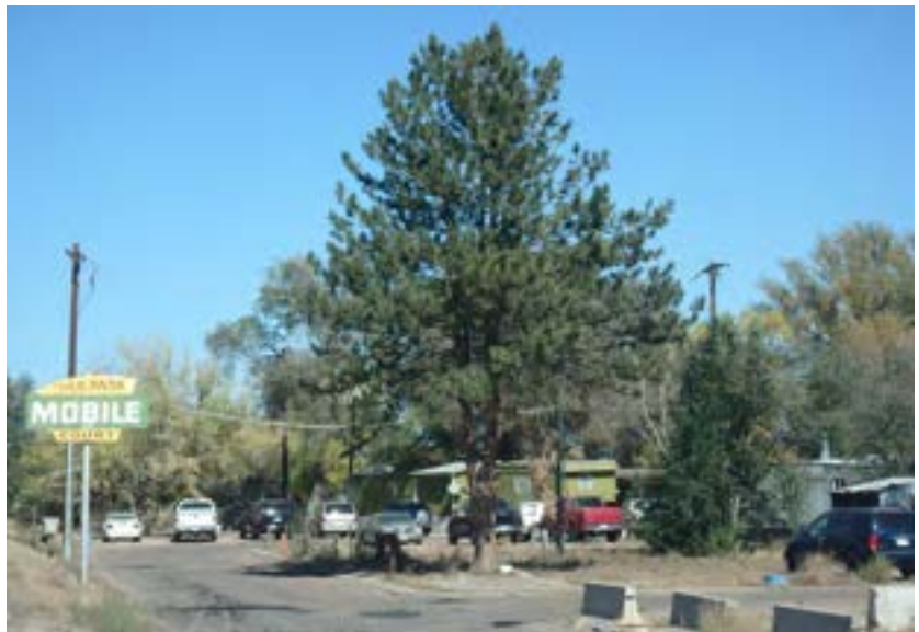
Figure 87. River Park Mobile Court, 542 N. 11th Avenue. This mobile home park was constructed prior to 1967 as visually evidenced by its sign.
