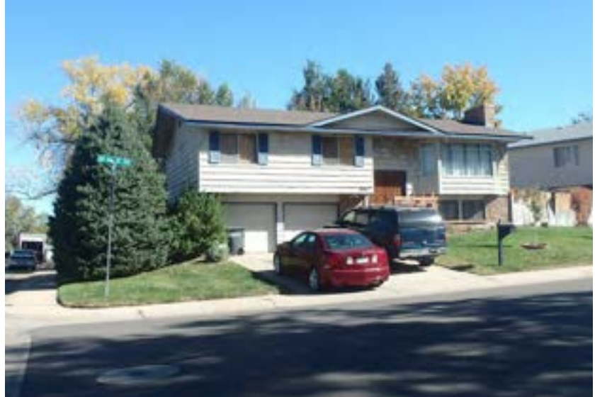
Figure 90. 1841 26th Avenue Place. This Bi-Level Split shows the stacked lower “noisy” level and upper “quiet” level with a central entry.
