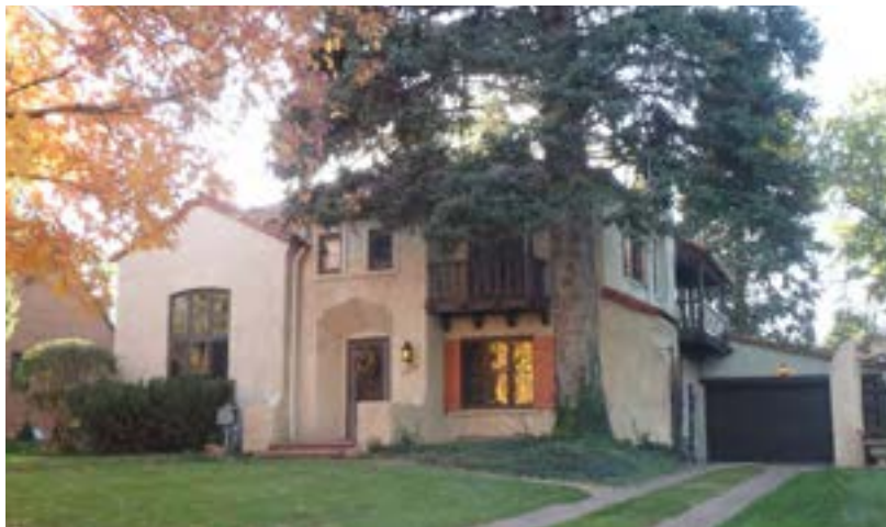
Figure 102. Bier House, 1919 14th Avenue. This residence was constructed by Contractor Otto F. Stoffgren in 1932 (Waldo 2016:105). Although its red tile roof, and stucco cladding help to identify it as a Spanish Revival or Mediterranean Revival style residence, its decorative arched portal, ornamental tablet, and wrought iron work help to mark it as a Spanish Revival residence, likely responding to the contemporary glamor of the Hollywood cinema (Gowans 1986:109).
