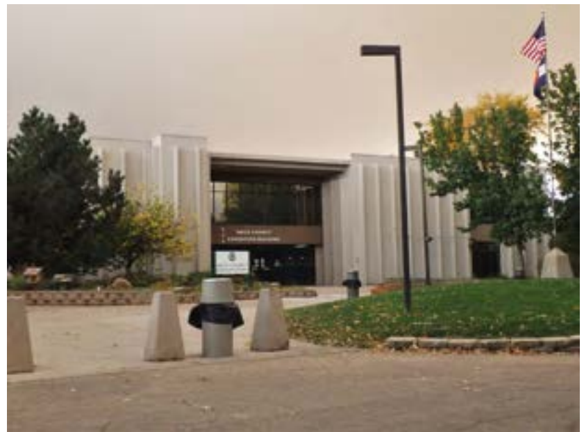
Figure 73. Weld County Exhibition Building, 525 North 15th Avenue. Public building showing the use of precast concrete double tees as wall elements.
