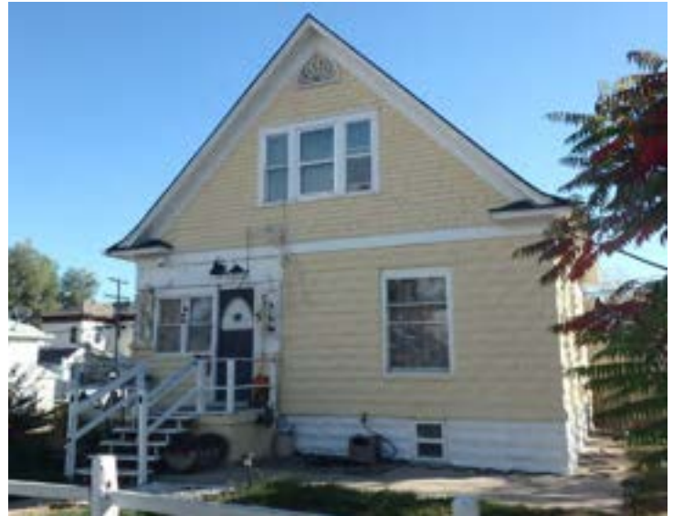
Figure 71. Gurney Residence, 1444 7th Street (5WL.602). Residence with a basement and ground story constructed from rockfaced concrete block masonry. The garage behind the building and residence east of it are also constructed from concrete block.
