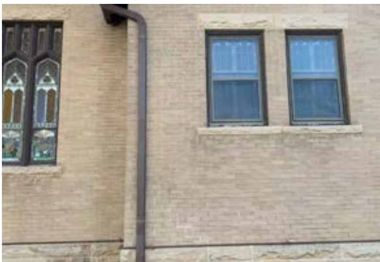
Figure 70. Saint Patrick Presbyterian Church (Old Park Church), 803 10th Avenue (5WL.928). Detail of north elevation showing a more refined buff colored pressed brick used for a street-facing wall of a high-status building.
