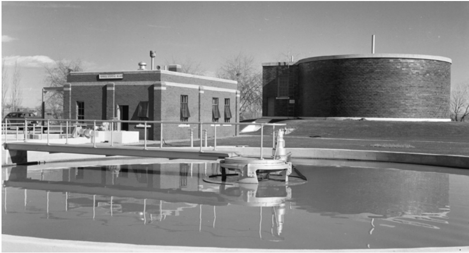
Figure 43. Historic photo of PWA-funded Greeley Sewage Disposal Plant. Sewage treatment plants were an important component of the PWA's legacy. Their construction helped dramatically to improve the public health of Coloradans who suffered from a numerous waterborne diseases which made the state among the unhealthiest in the West (Wolfenbarger 2005:E.52). 88.442.439, History Colorado. ca. 1935-1950. R. G. (Bob) Zellers.
