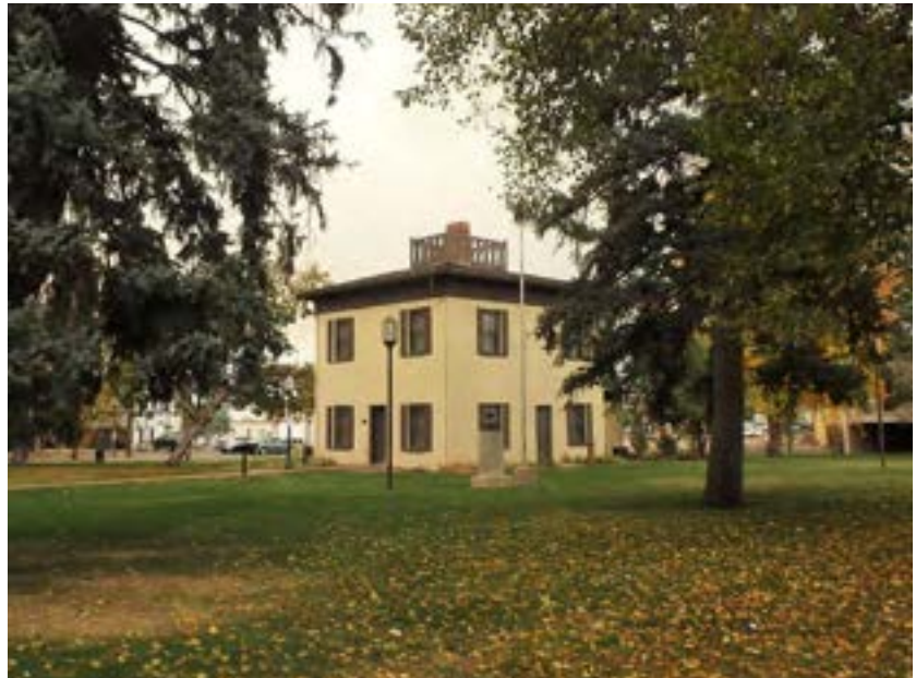
Figure 66. N.C. Meeker Home (Meeker Home Museum), 1324 9th Avenue (5WL.566). This unusual two-story adobe residence was constructed in 1870 in the Italianate style. It underwent several changes before a 1959 restoration returned it to its 1870s appearance (Fink 1970). Note the wooden balustrade atop the hipped roof which approximates the central tower of the American Italianate style.
