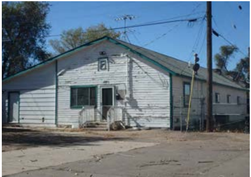
Figure 67. 1521 North 25th Avenue. An example of vernacular wood-frame construction with wood cladding in the Espanola Subdivision, colloquially referred to as "Spanish Colony."
