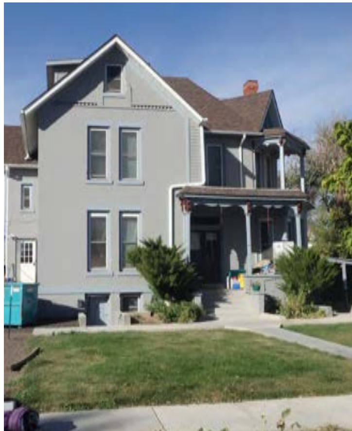
Figure 7. Robert Hale House, 1421 8th Street (5WL.575). The Robert Hale House was determined both individually eligible and eligible as a contributing resource to a historic district for NRHP listing in 1981. The age of this determination is such that a new determination will likely have to be made before this property can be designated.
