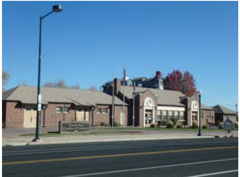
Figure 62. Union Pacific Depot, 902 7th Avenue (5WL.764). This building is significant for a number of reasons including its prominent architect Gilbert Stanley Underwood, as well as its association with Greeley's development and the maturation of its rail line.
