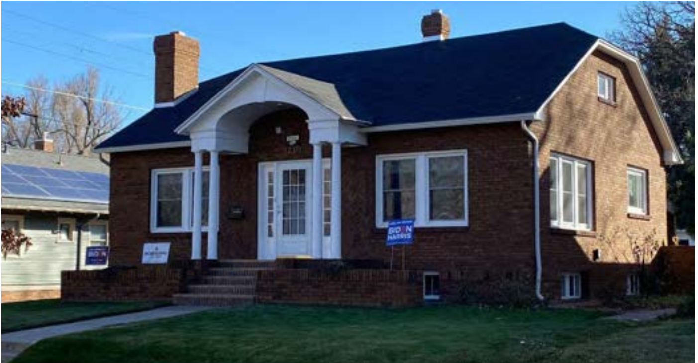
Figure 40. 1218 Cranford Place. View showing a small side gabled bungalow with jerkinheads and a classically-detailed entry. Although not identical to Figures 41a & b, this residence shows similarities in its form and detailing and may stem from another catalog publisher, nearly all of whom provided models of single-story jerkin-headed classical bungalow for sale (Antique Home Style n.d.). Courtesy of Scott McLean. November 2020.
