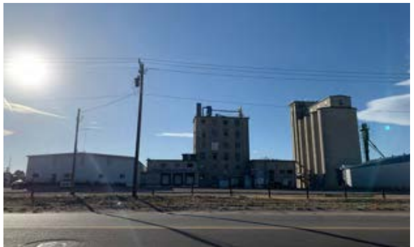
Figure 54. Trinidad Bean & Elevator Company, 615 5th Street. This collection of buildings may also form part of a cultural landscape which showcases the manner in which agricultural products were stored and transferred between rail and road vehicles.
