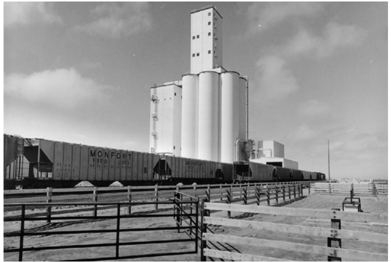
Figure 44. Monfort feedlot near Greeley shown sometime after the construction of feed storage silos in 1946. 90.447.26, History Colorado. ca. 1940-1960. James L. Ehernberger (uncertain).
