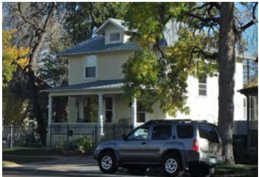
Figure 85. 1326 8th Street. This house is an archetypical example of a Foursquare with its square plan, two-story height, full-width porch, hipped roof, and single dormer.
