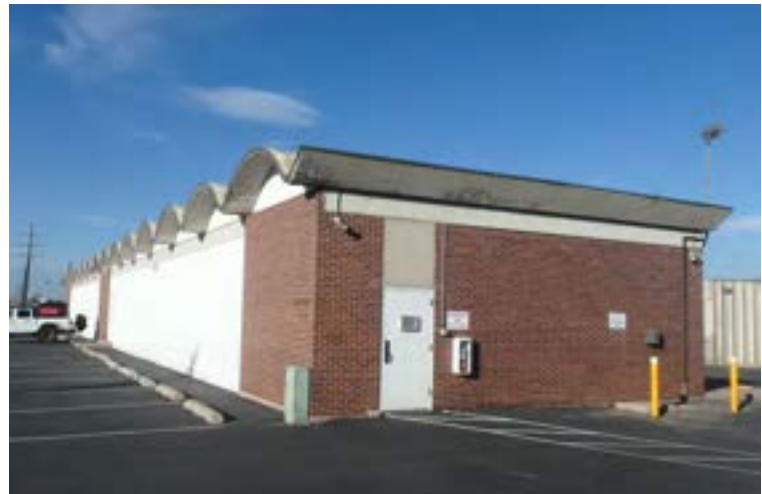
Figure 48. Hensel Phelps Construction Co., Building 2, 420 6th Avenue. This storage warehouse with a remarkable undulated thin-shell concrete roof was constructed in 1961 according to data from the Weld County Property Portal.
