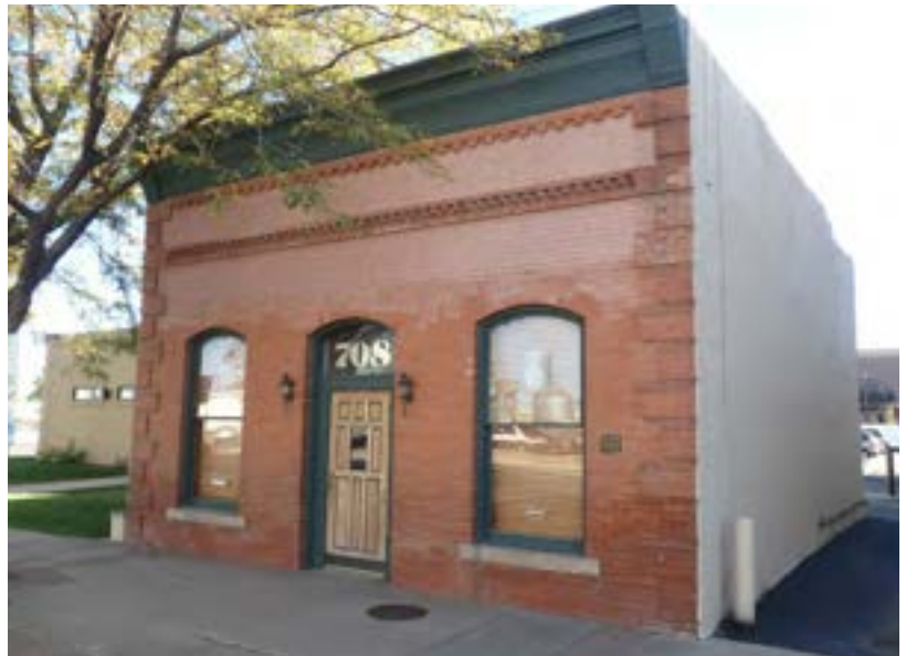
Figure 78. New Cache la Poudre Irrigation Company Building, 708 8th Street (5WL.2576). This 1902 One-Part Commercial Block is distinguished by its single-story brick masonry construction, orientation to the street, and decorative, stamped tin cornice.
