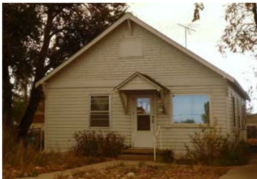
Figure 75. 424 11th Street. This residence is an example of a Gable-Front, with its clearly articulated single gable roof facing the street. Craftsman detailing is visible with the knee braces and use of multiple types of wall cladding.
