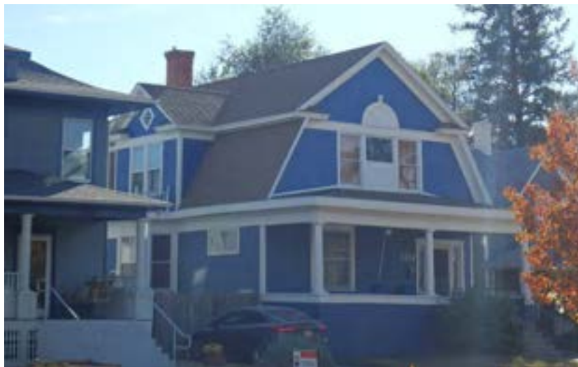
Figure 101. 1214 8th Street. Archetypical example of a Dutch Colonial Revival showing its characteristic gambrel roof and classical detailing.
