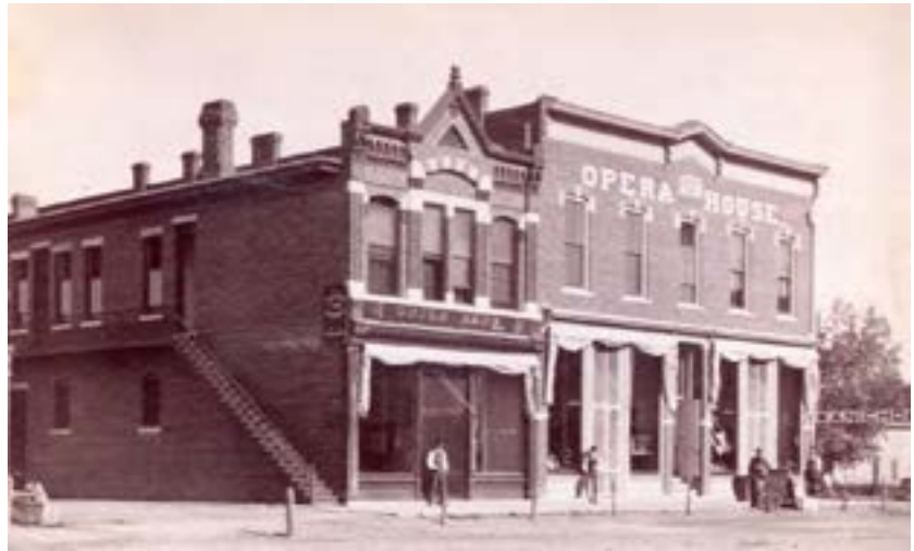
Figure 95. Although no longer extant, both buildings once located in downtown Greeley are good examples of the Nineteenth Century Commercial style with ground story display windows, upper sash windows, and high parapets all decorated by an eclectic mix of ornamentation. (WHJ-10152, Denver Public Library Western History and Genealogy Dept., Denver Public Library).
