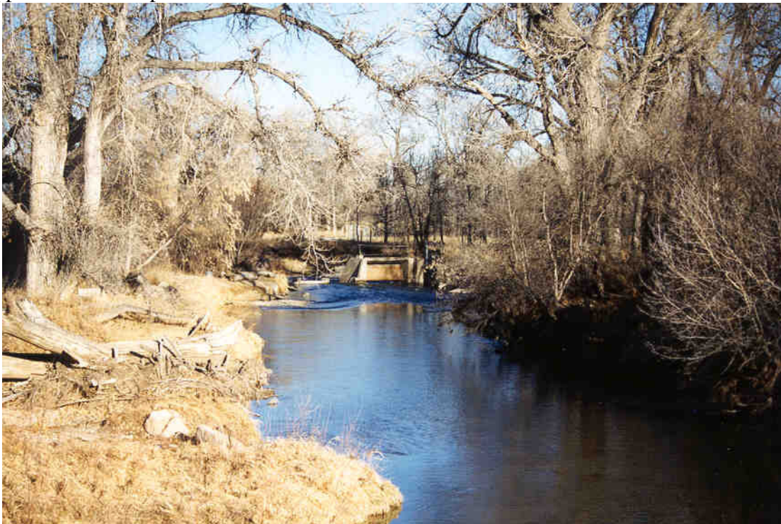
Jones Ditch Dam and Headgate
