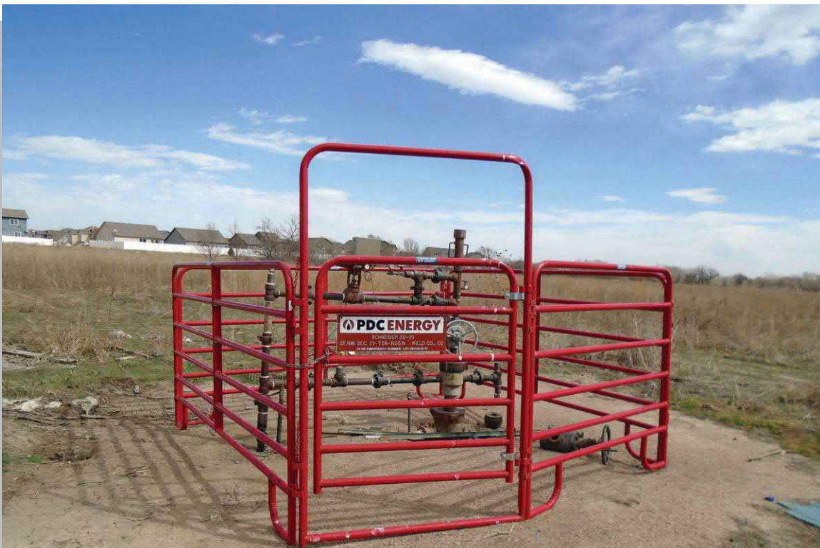
Photo 10 - The Schneider #22-21 oil and gas wellhead on the property.
