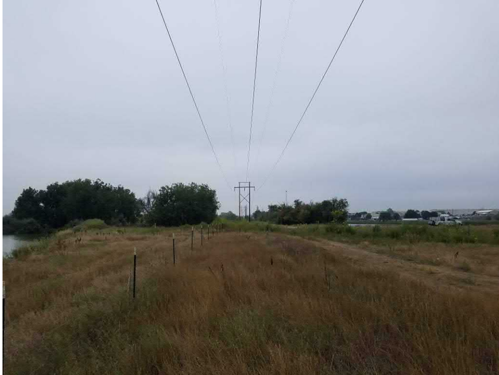
Photo #11 View of 5WL.3155.1. View to the west.
