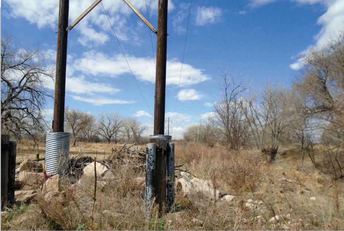
Photo 7 - The high-voltage overhead powerline and concrete rubble used as erosion control.
