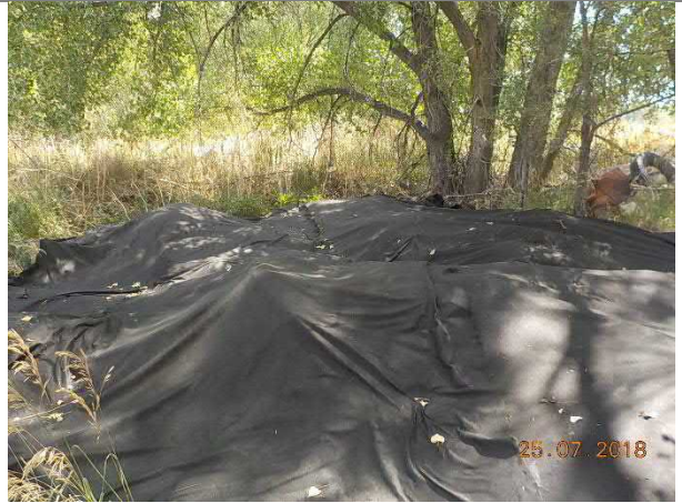
Photo #4 View of geotextile installed in I15-1
