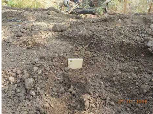
Photo #9 View of verification of 6+ inches of soil at H10-5
