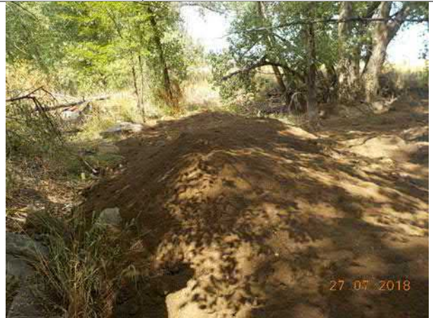
Photo #12 View of soil placement at I15-1
