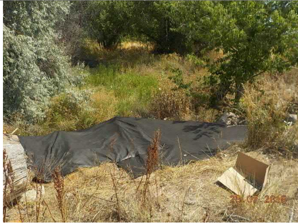
Photo #1 View of the geotextile installed in H10-5
