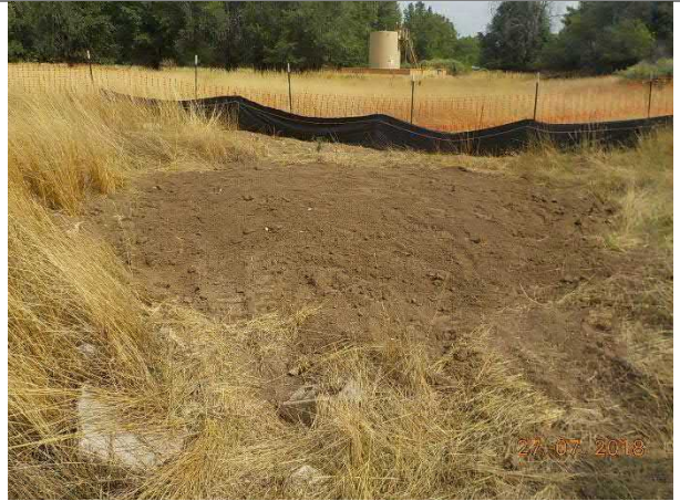
Photo #15 View of soil placement at O28-2
