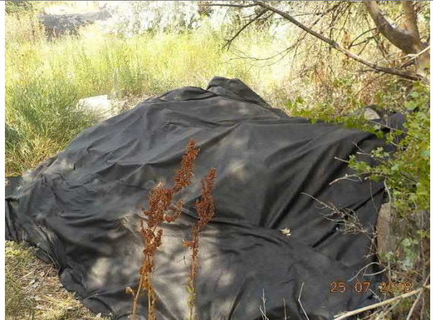
Photo #2 View of the geotextile installed in J17-2 and J17-3
