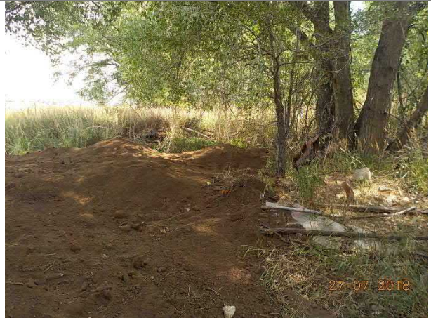
Photo #13 Second view of soil placement at I15-1
