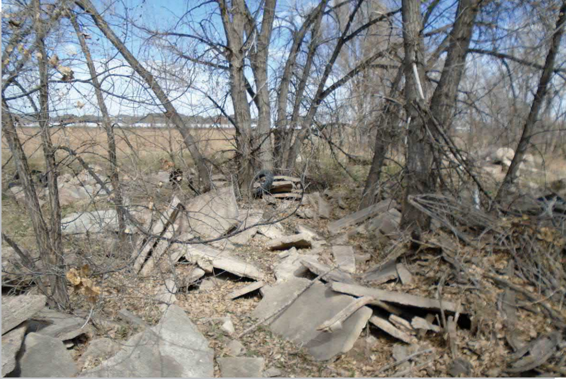
Photo 5 - Concrete debris observed on the property.
