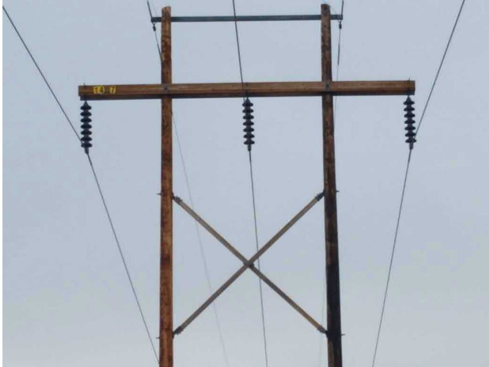
Photo #13 View of View of 5WL.3155.1, close-up. View to the east.
