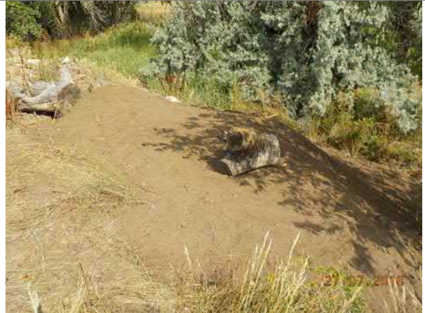
Photo #8 View of soil placement at H10-5
