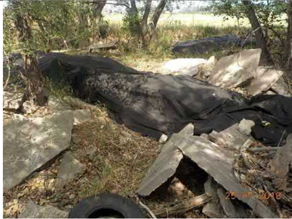
Photo #3 View of the geotextile installed in I15-1
