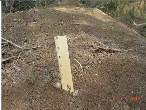
Photo #11 View of verification of 6+ inches of soil at J17-2 & J17-3
