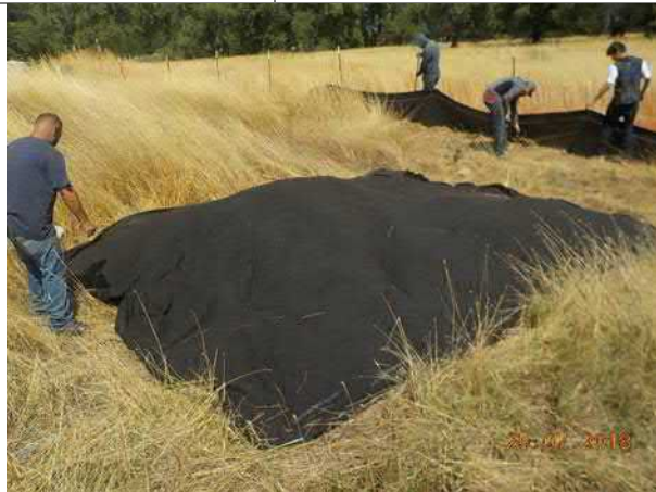
Photo #5 View of the geotextile installed in O28-2
