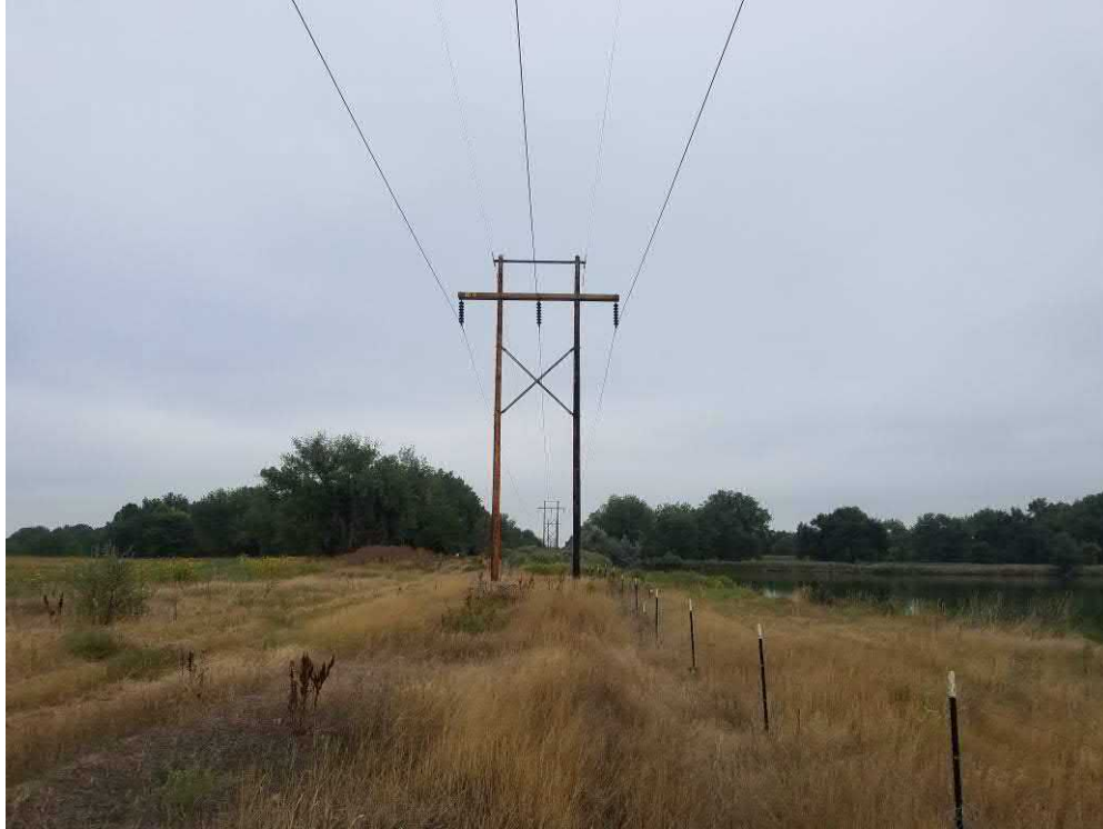
Photo #12 View of 5WL.3155.1. View to the east.
