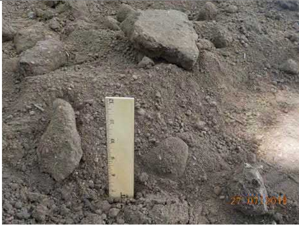
Photo #14 Second view of soil placement at I15-1
