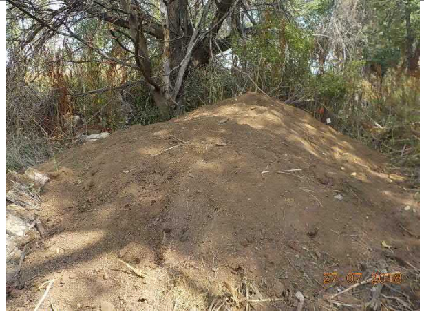
Photo #10 View of soil placement at J17-2 & J17-3
