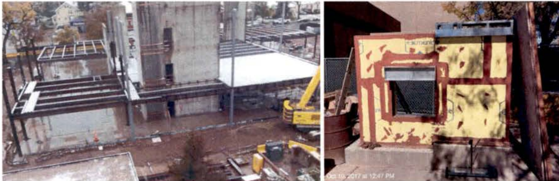
View from Wemcam on top of Annex Bldg, Mock-up of wall systems
