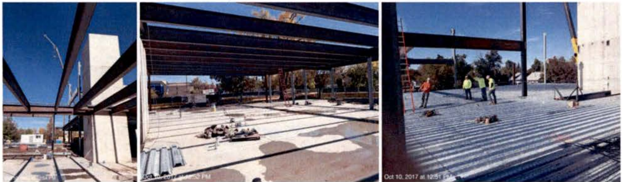
View from inside the courtroom looking North, and East, @nd level metal decking installation
