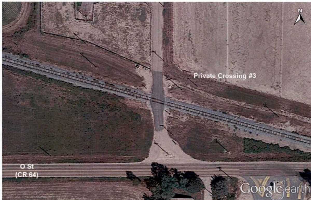
Figure 15. Private Crossing #3 - Aerial View
