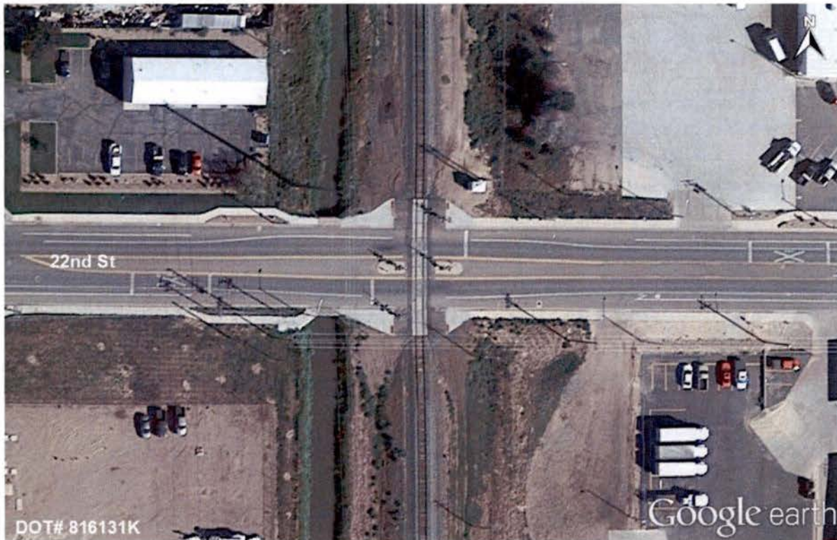
Figure 9. 22 nd Street - Aerial View
