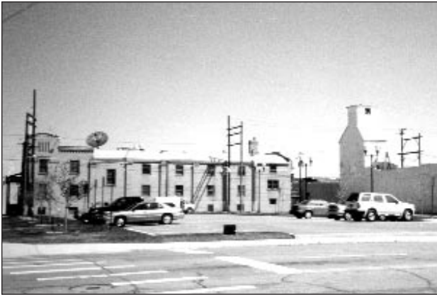
Where there were once historic commercial buildings in downtown Greeley, there are now parking lots. These are potential redevelopment sites
