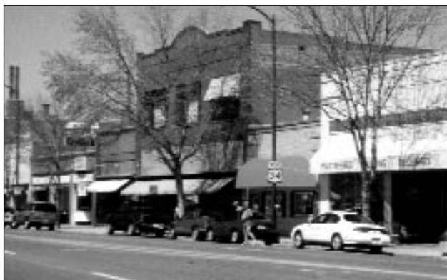
Brick commercial buildings with detailing at cornices, windows and entries
