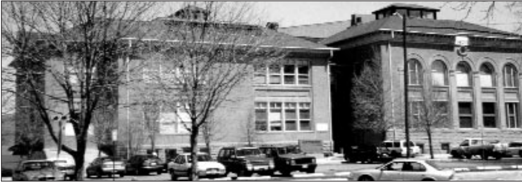
Greeley High School (no longer in school use) is a civic building of more than two stories in height
