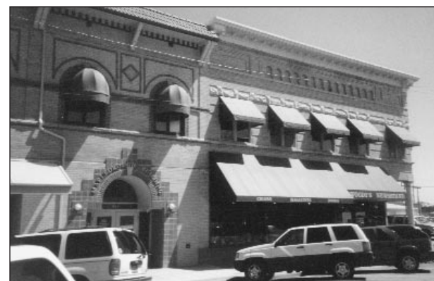
Examples of architectural detailing of historic buildings
