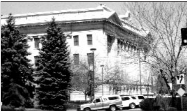
Secondary facade of a civic building
