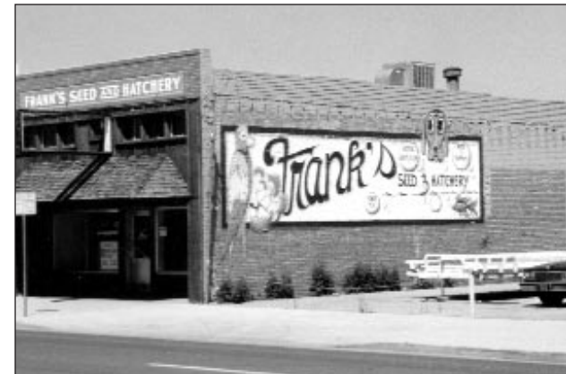
Signs painted on brick walls were common on historic buildings
