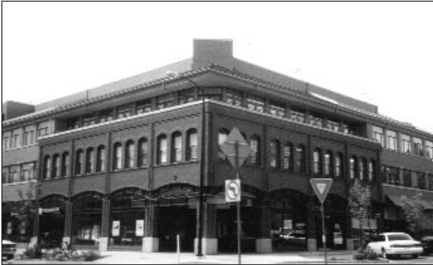
Parking structure with commercial/office space wrap on one-quarter block
