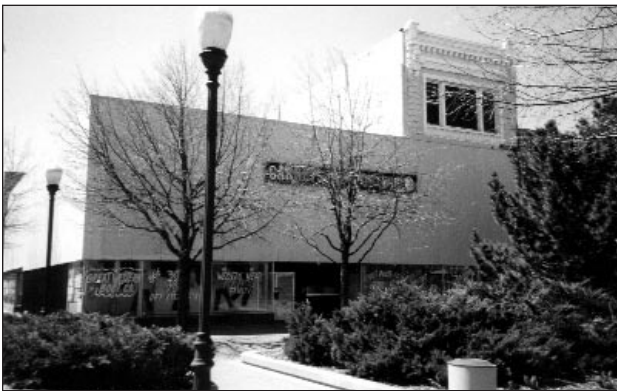
Historic details have been covered over
