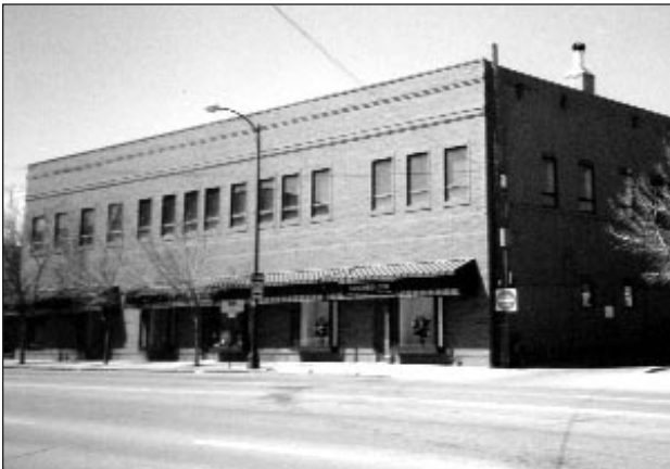
New building incorporates the pattern of primary and secondary facades typical of historic buildings in the area
