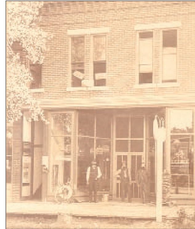
City of Greeley Museums - Permanent Collection Typical historic storefront
