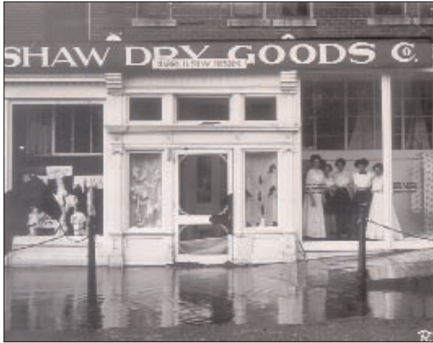
City of Greeley Museums - Hazel E. Johnson Collection Pattern and detail of historic windows and doors
