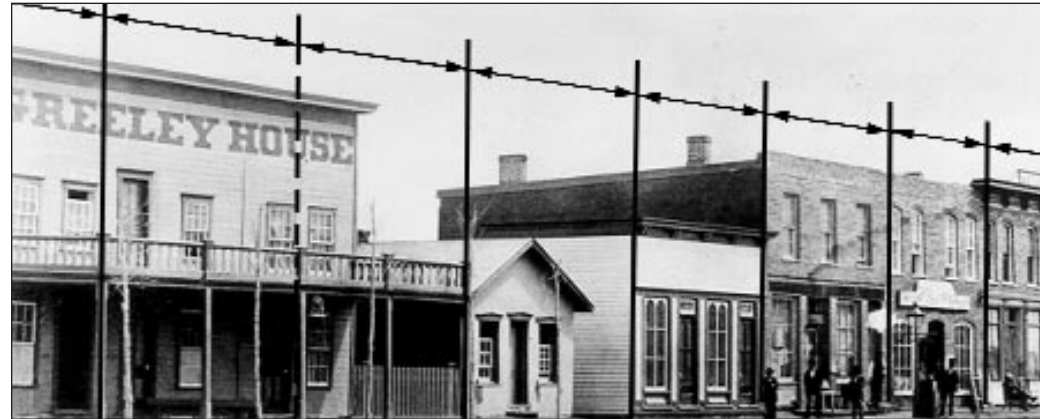
Horizontal alignment of historic building elements
