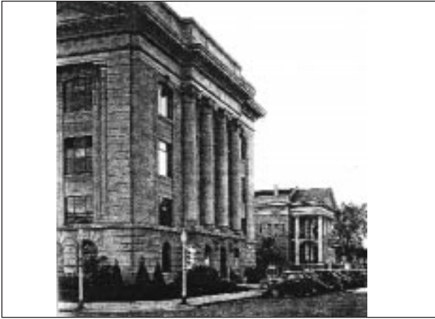
Weld County Courthouse - 9th Avenue and 9th Street - built 1915 Source: City of Greeley Museums - Permanent Collection
