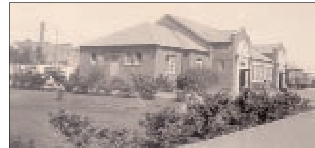
Greeley Union Pacific Depot - 902 7th Avenue - photo 1930’s
