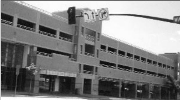
Parking structure without wrap; incorporates some characteristics of historic buildings
