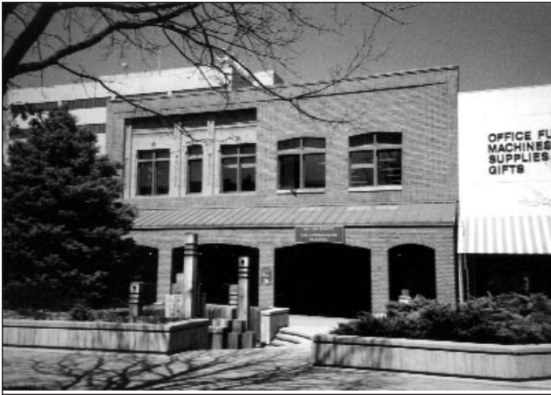
Altered facade of historic commercial building
