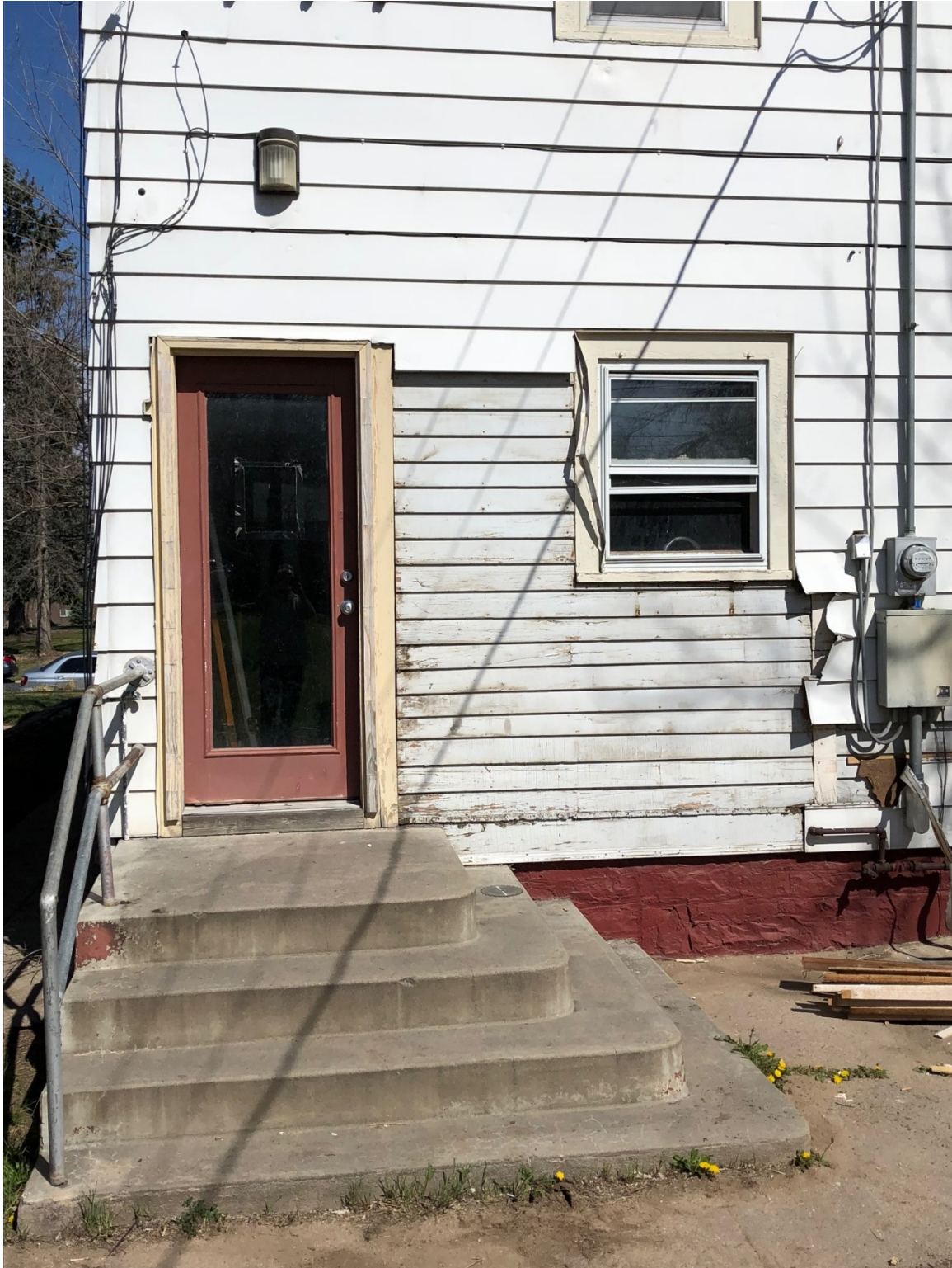
Original wood lap siding under metal siding
