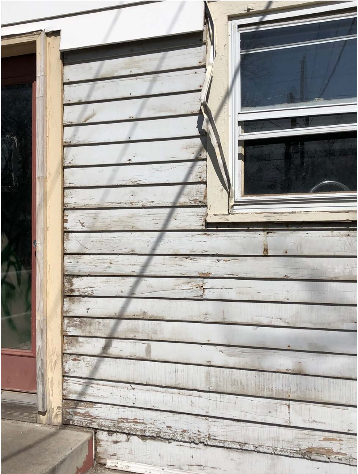
Original siding under metal siding on rear April 2018
