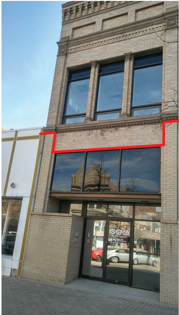
PHOTO SHOWING AREA OF BUILDING AT NEW ATM. EXISTING TAN BRICK AT FACE OF BUILDING WOULD REMAIN. THE BRICK THAT IS BELOW THE RED LINE IS NOT ORIGINAL. STOREFRONT IS ANODIZED BRONZED ALUMINUM. TAKEN: MARCH 22, 2019
