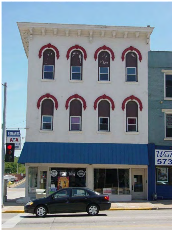
A recent window and facade "Upgrade".
