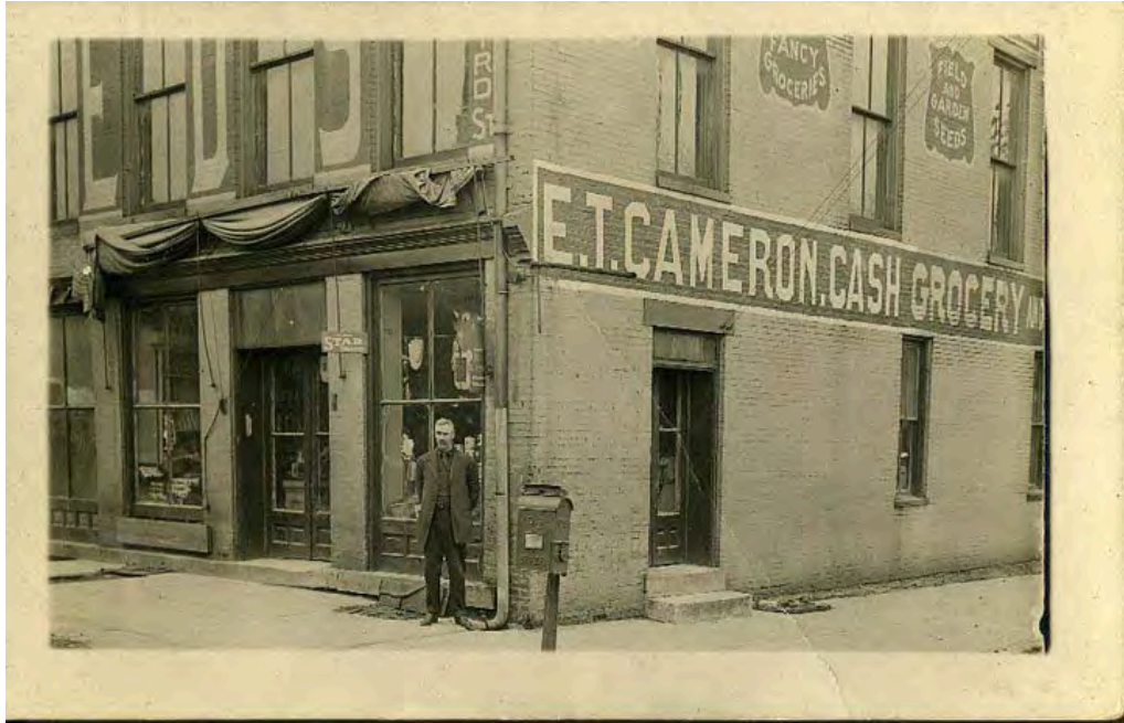
1910 Main Street building with retractable awnings
