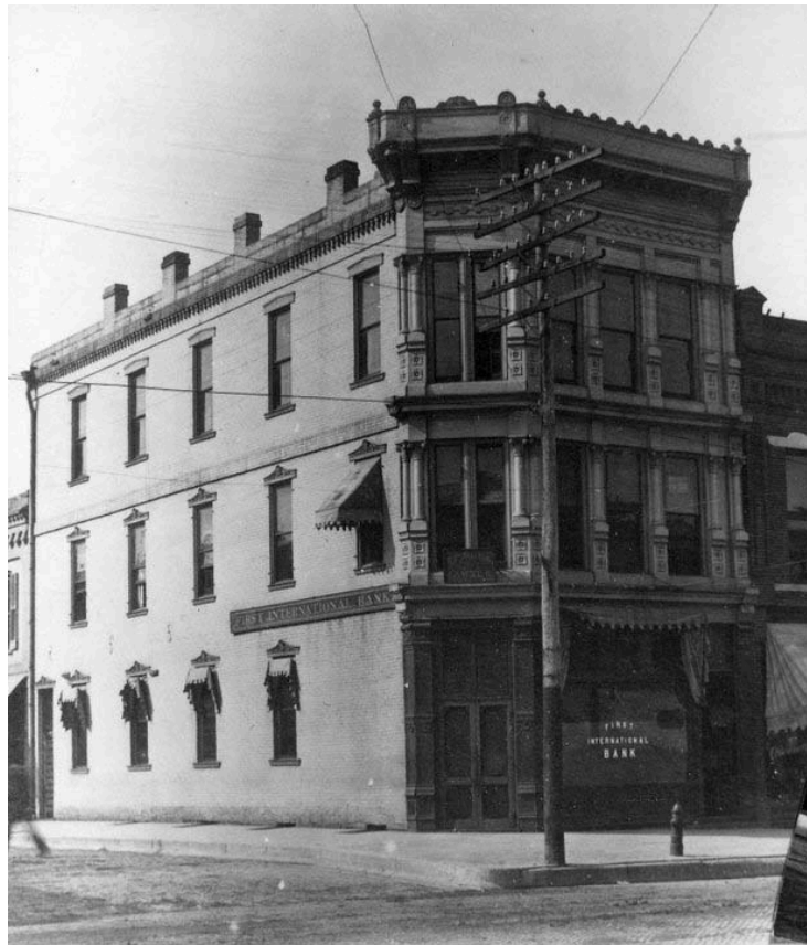
1904 Main Street building with retractable awnings
