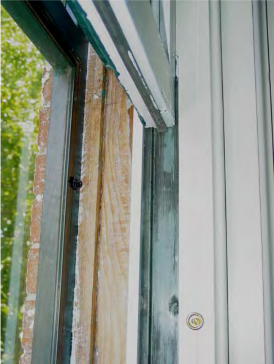
Metal track, rubber gasket & removable storm panel. Less air infiltration than a replacement window
