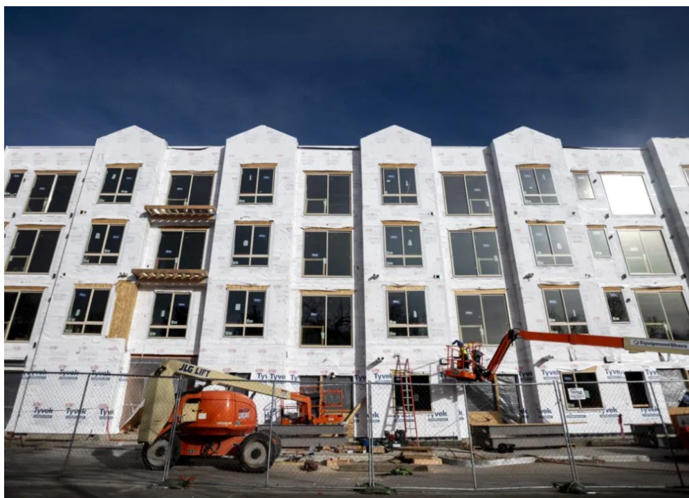
Construction workers work on the Boone at Maddie apartment complex under construction on 8th Avenue between downtown and the University of Northern Colorado in Greeley Tuesday, Nov. 19, 2019. (Alex McIntyre/amcintyre@greeleytribune.com)
