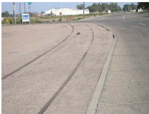
Rails Intersecting Private Property and Rails Running into Roadway/Intersection
