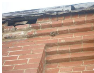
Deteriorated Gutters and Bldg.
