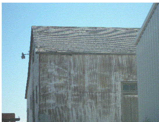
Deteriorated Tin Exterior and Roof (Sugar Factory)
