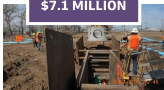
North Greeley Sewer Phase 2A
