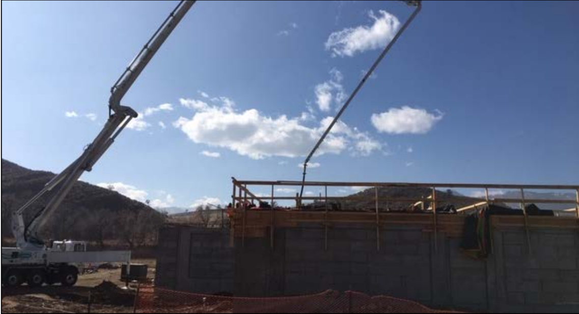
WTP Concrete Floor Being Poured
