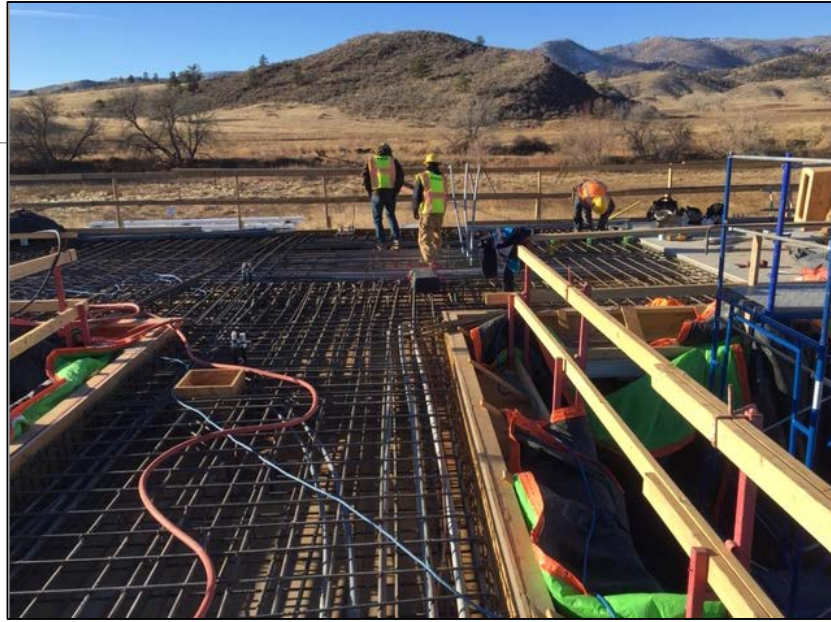
Rebar for Operating Floor
