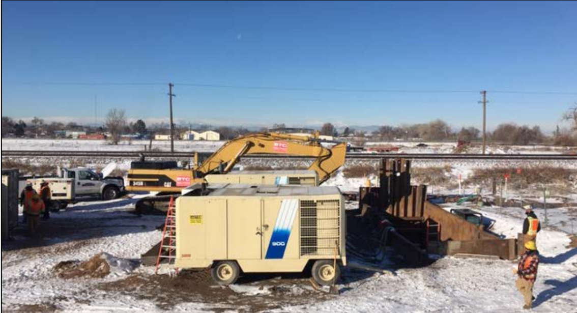
Boring Pit UPRR
