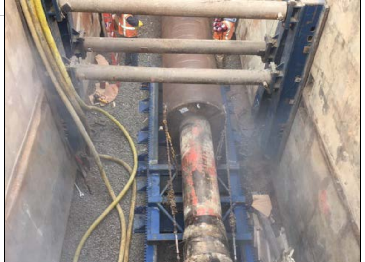
Boring Shaft UPRR Guided Pipe Hammer
