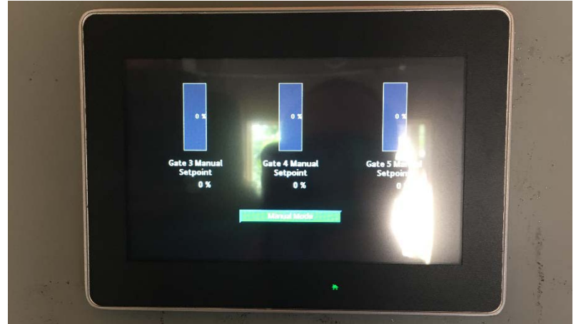
New SCADA Controls at Lake Loveland
