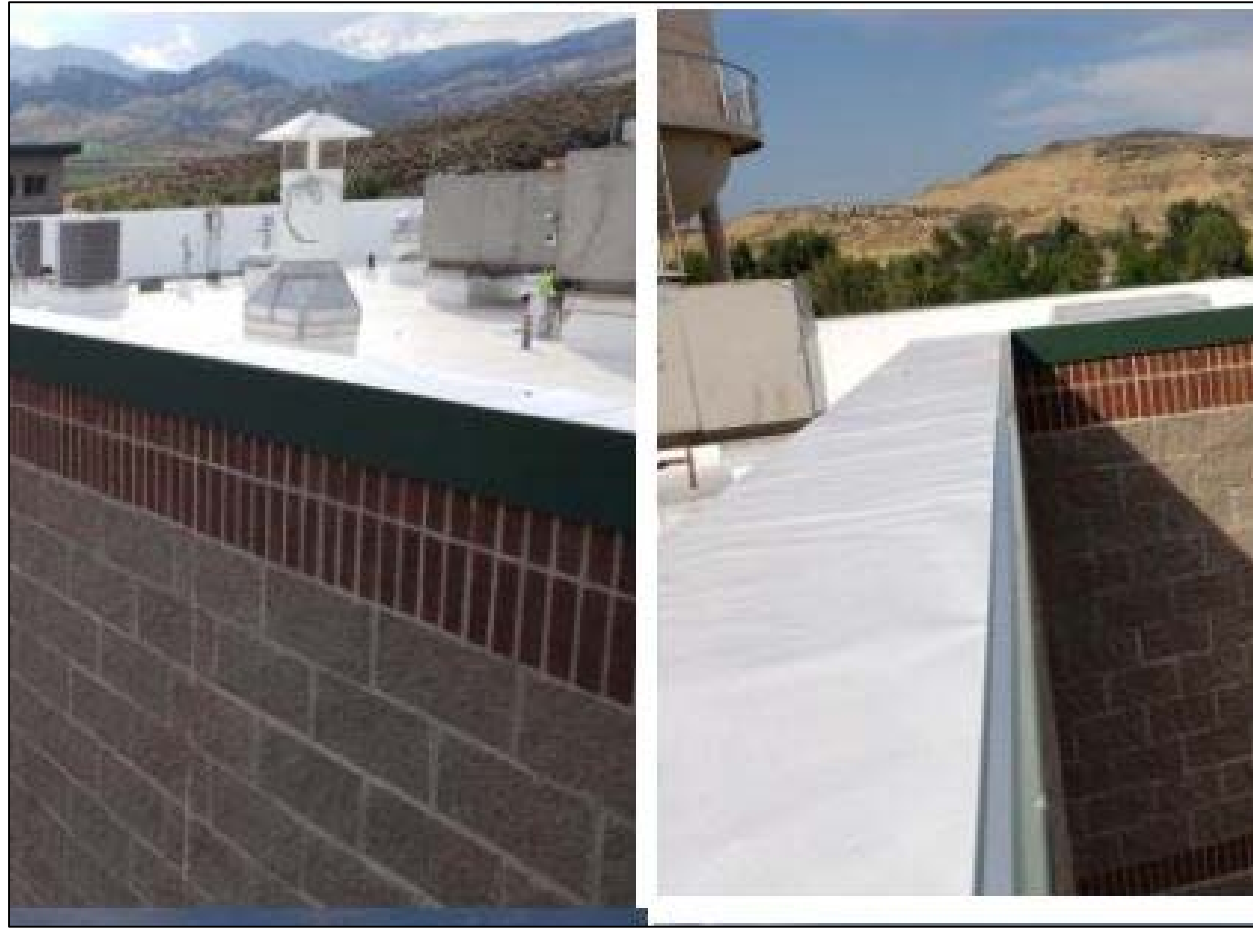
Building Roof Replacement
