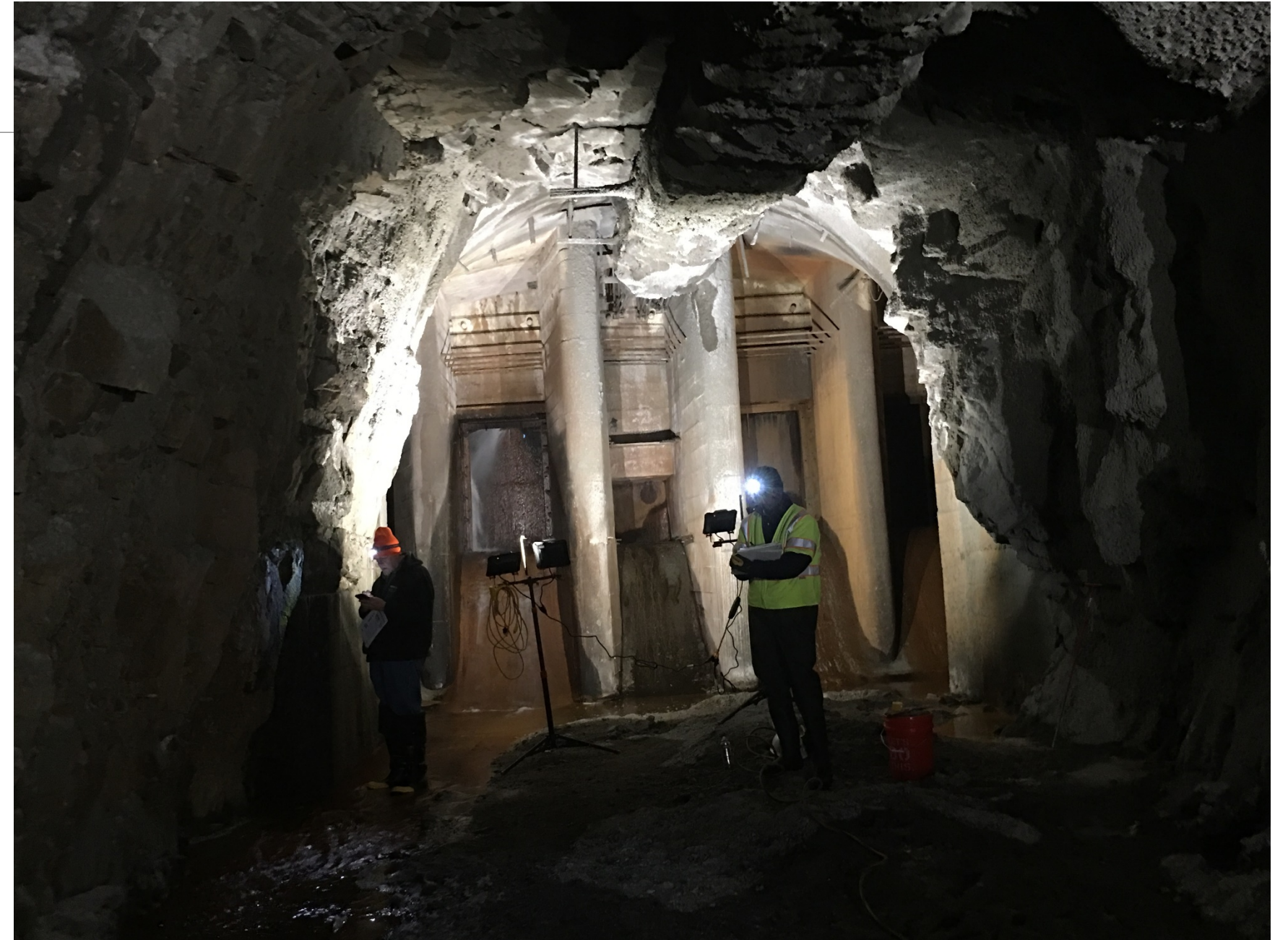
Existing Gates at Bottom of Reservoir
