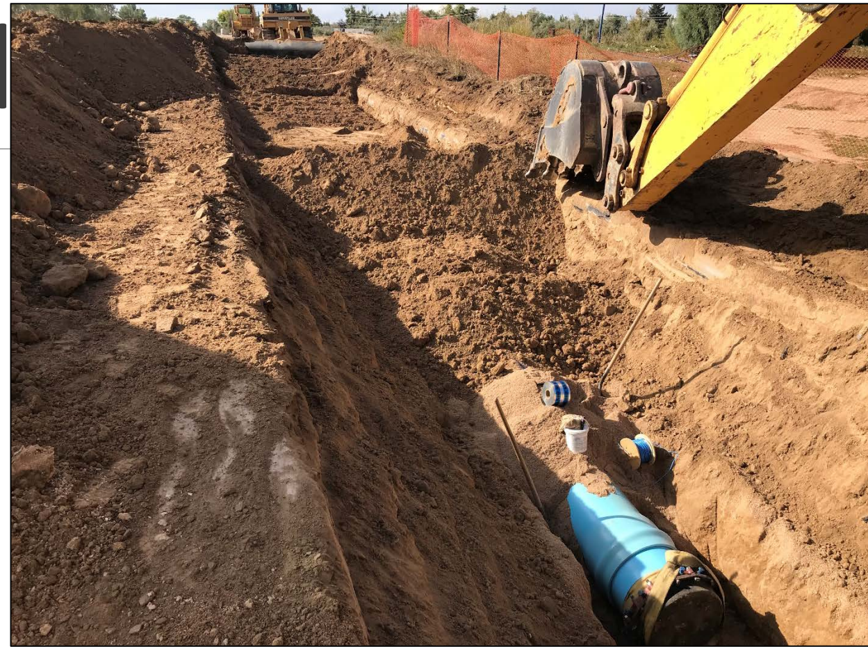
New Pipeline Segment
