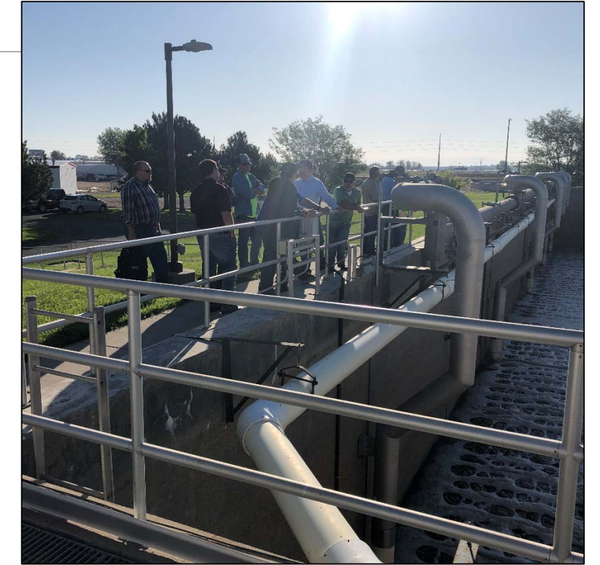
On Going Electrical and SCADA System Replacement
