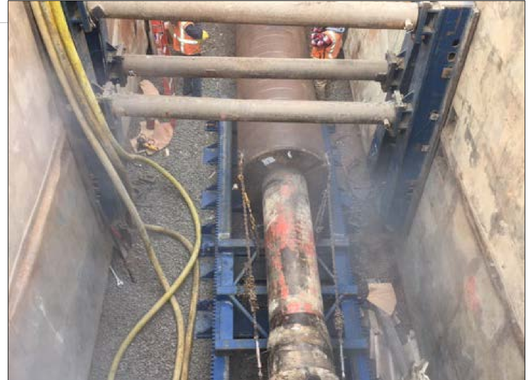
Boring Shaft UPRR Guided Pipe Hammer
