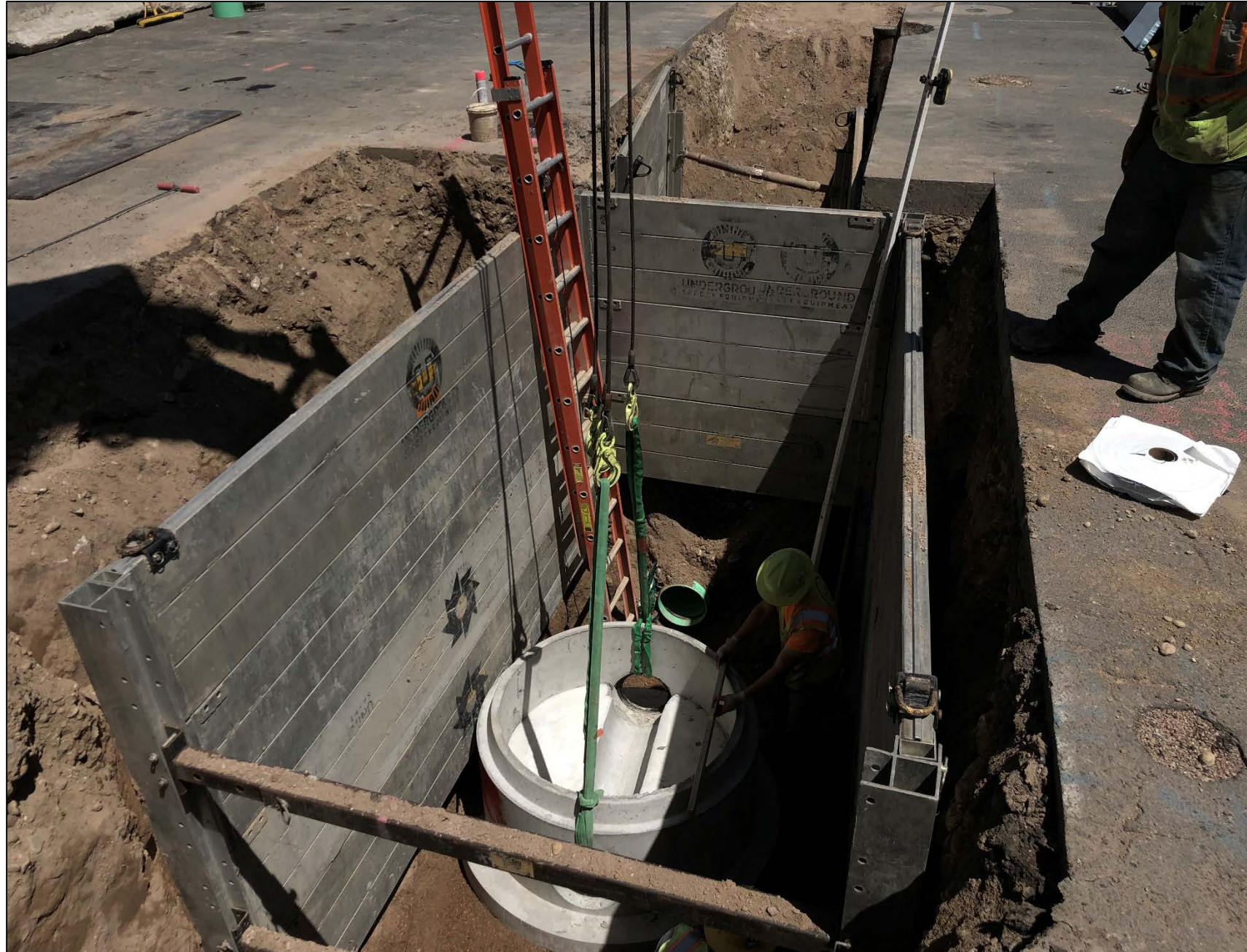
New sewer line manhole installation
