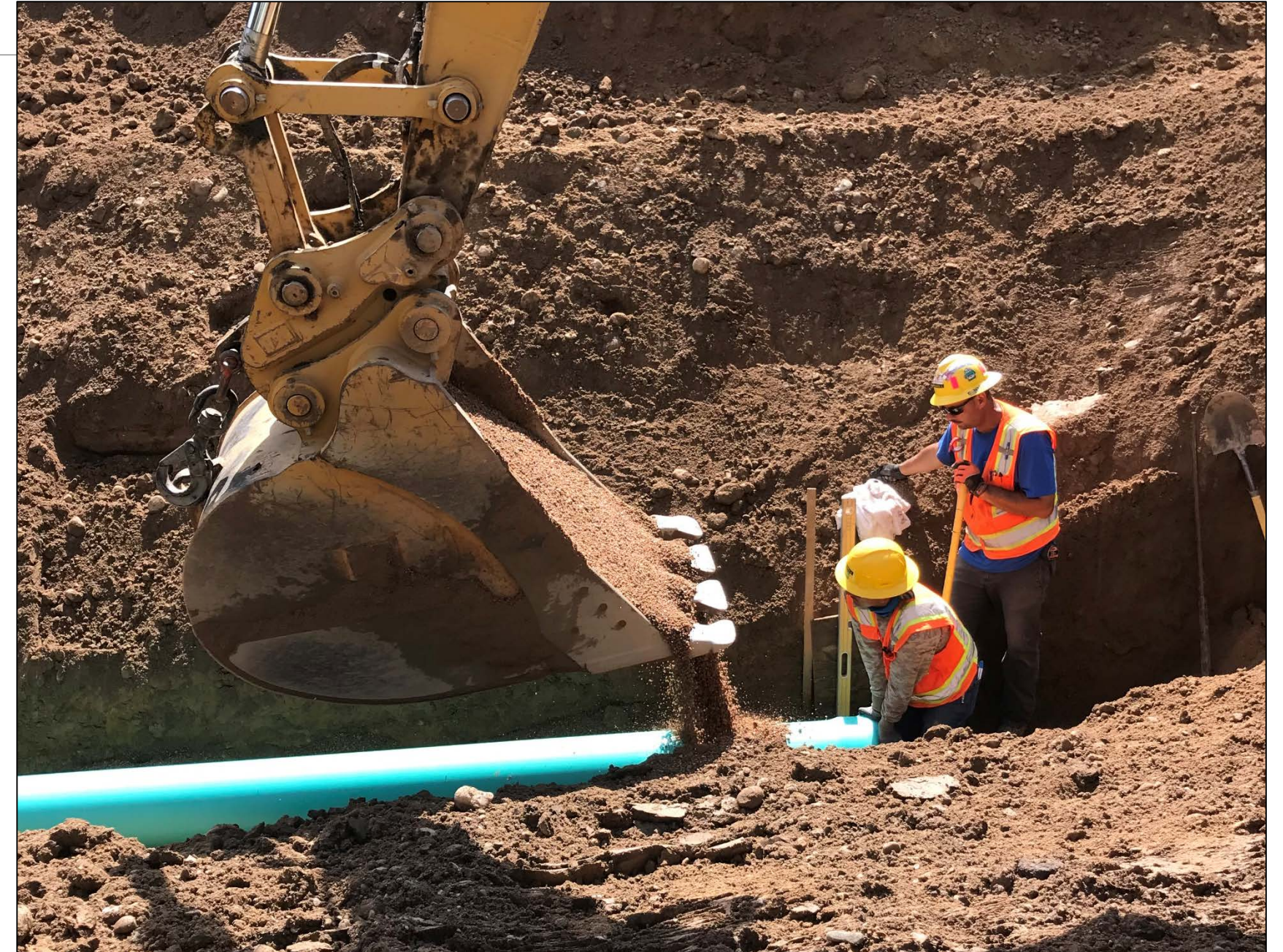
New water main installation
