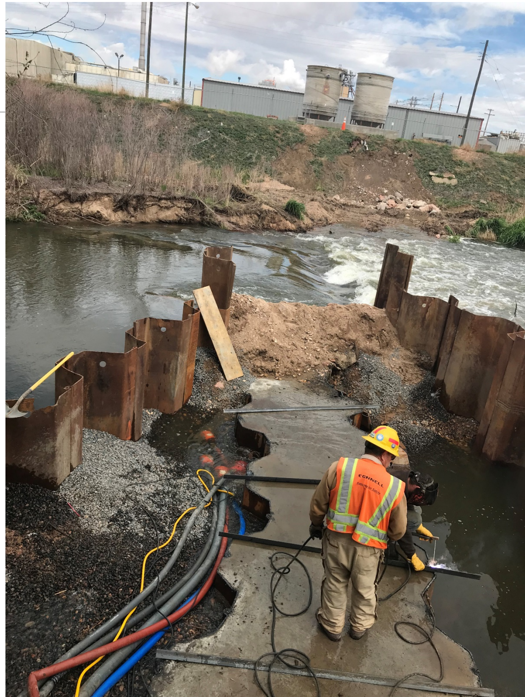
Construction of Sewer Protection
