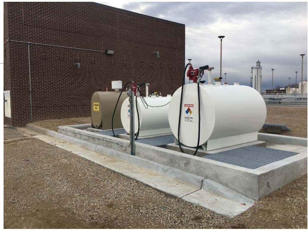
New Fuel Station
