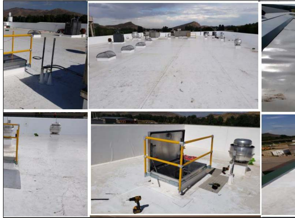
Chemical Building Roof Replacement
