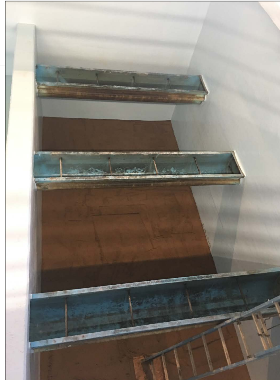
Finished Sand Installation
