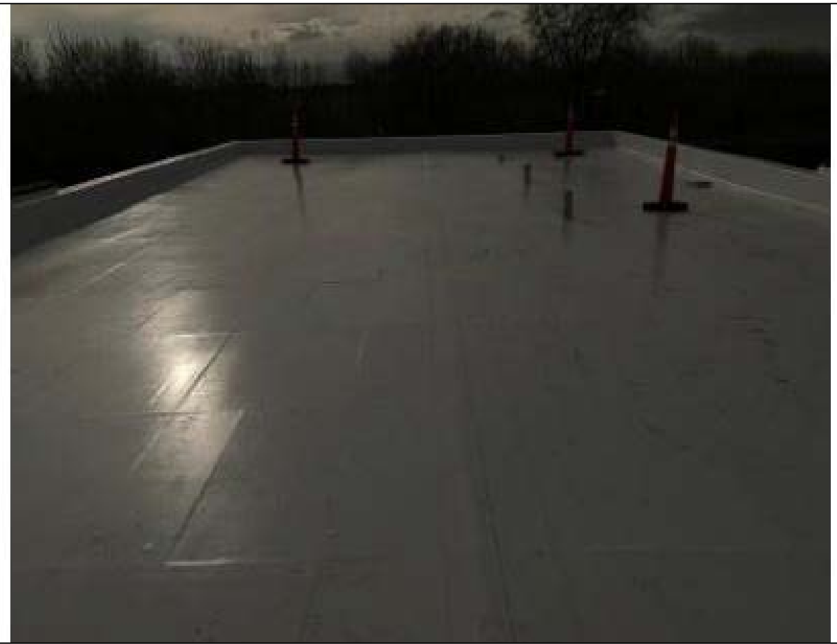
Filter Building Roof Replacement
