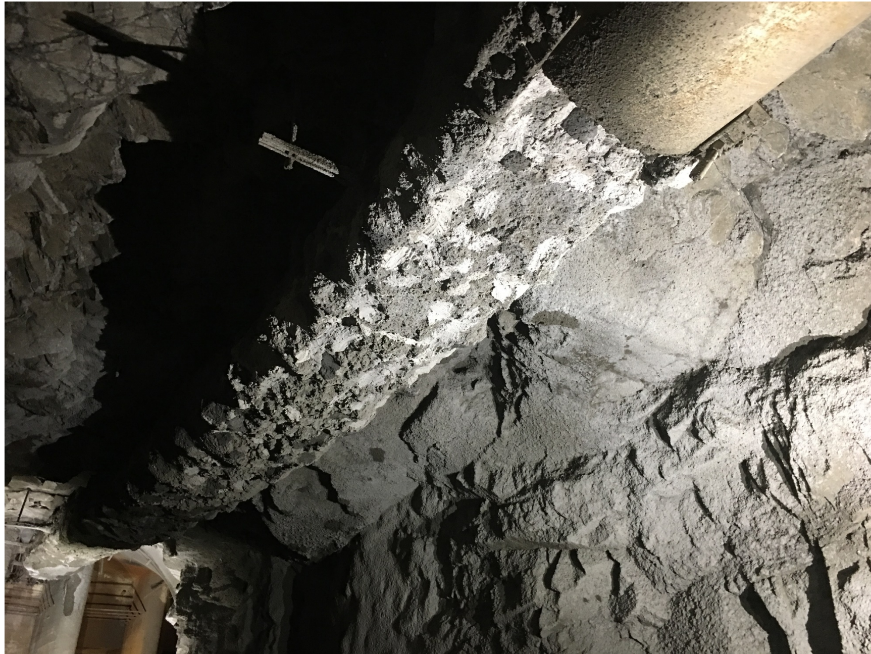
Shotcrete Protection of Hydraulic Lines
