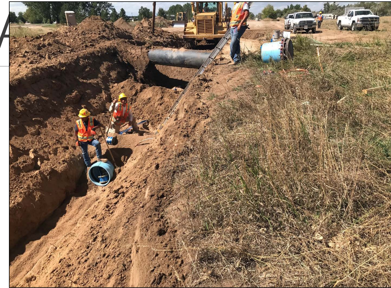
PVC Pipe Installation
