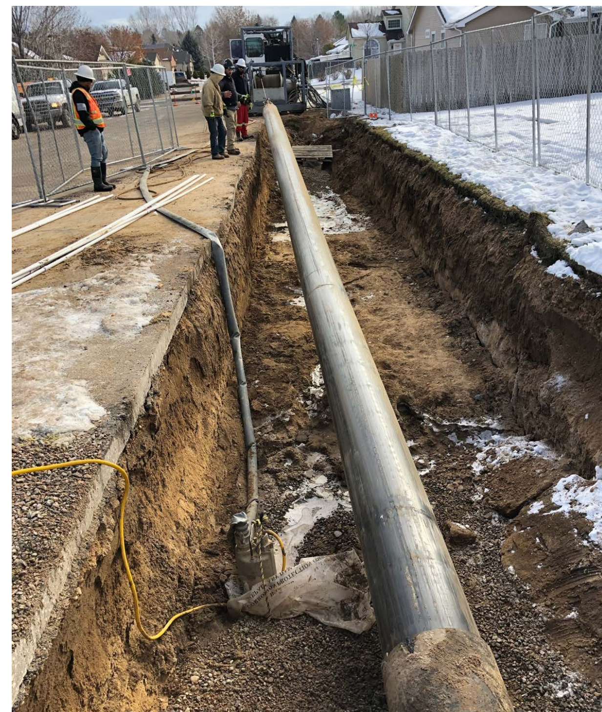
Lining a Pipe Segment
