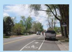
Figure 3-18: 13th Street after right sizing
